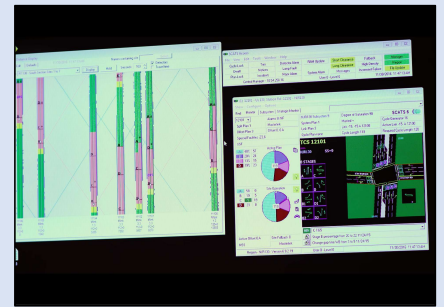
Intelligent Traffic Signals
