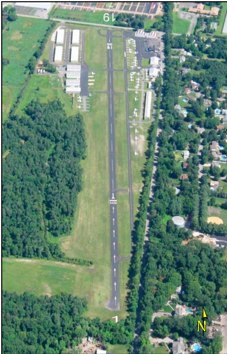
Lincoln Park Airport (N07) Lincoln Park, NJ
