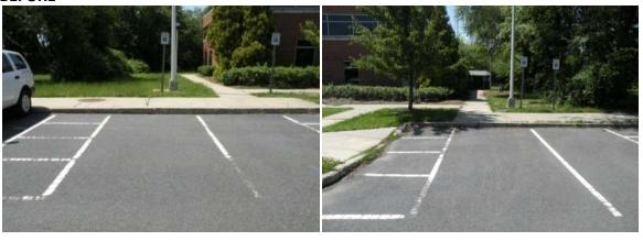
AFTER: Parking spaces were restriped and handicap parking spaces marked with the International Symbol of Accessibility (handicapped symbol). Two (2) spaces were eliminated along the front of the building on each side to meet 8 foot wide access aisle requirements. Work completed 9/13/10.
