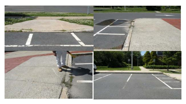
AFTER: Installed (4) new Curb Ramps (9/13/10) and (4)Truncated Domes 9/20/10
