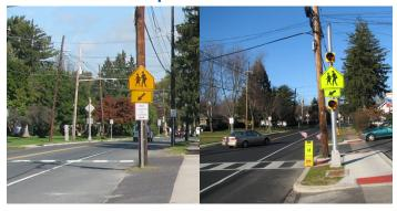
As an on-call traffic consultant for Lawrence Township, Arora designed improved pedestrian crossings at the intersection of Route 206 and Lawrence Avenue – Pilla Avenue. ADA-compatible, pedestrian ramps were installed on all corners and ladder-type crosswalk markings were installed at all crossings. Arora also designed new rectangular rapid flashing beacons for future installation at the Route 206 approaches.
