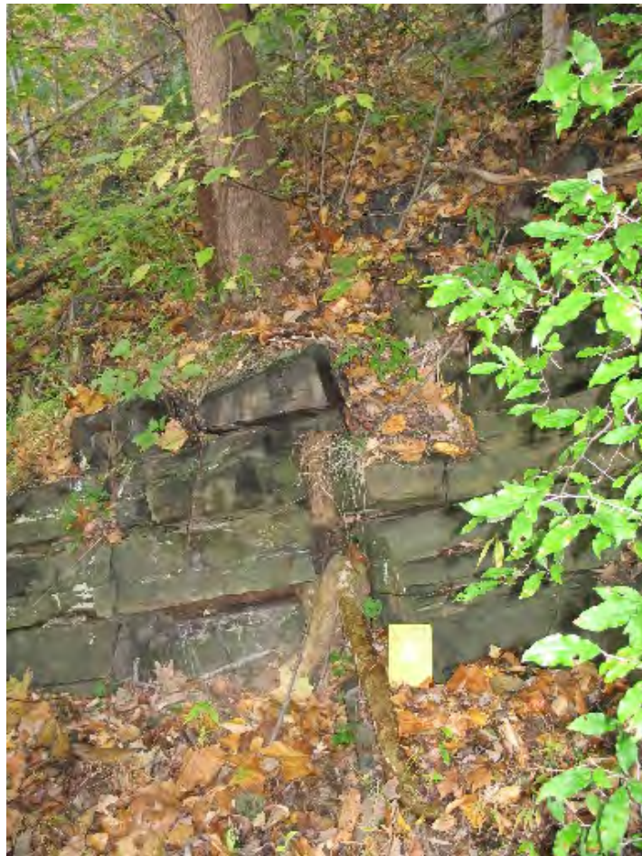
PHOTO 2 – Example of Root Wedging (Toe of Slope, Area D, Looking Northeast)
