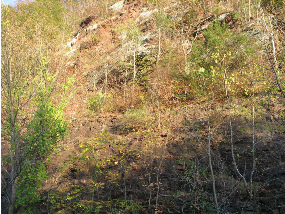
Photo 8 - Mid-Length of Area D, MP 30.08
