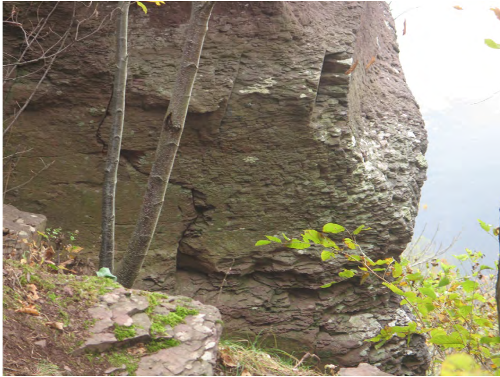
Photo 13 - S-shaped crack in North Side of Block above Devils Tea Table (Area D)
