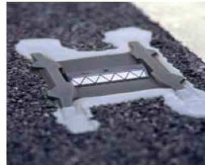
Snowplowable Raised Pavement Marker.
