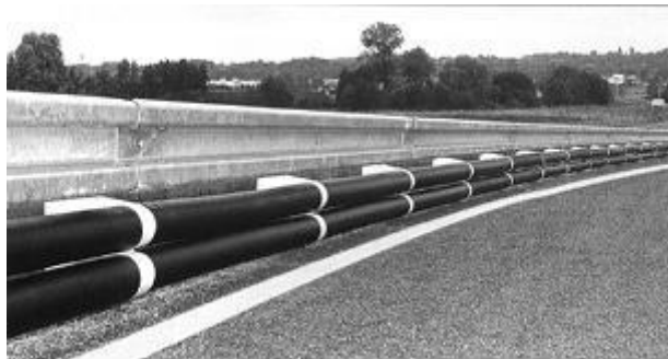
Figure 3. The Mototub by Sodirel. The Mototub is made from 70% recycled material and prevents motorcyclists from hitting the posts of the guardrail (FEMA, 2000).
