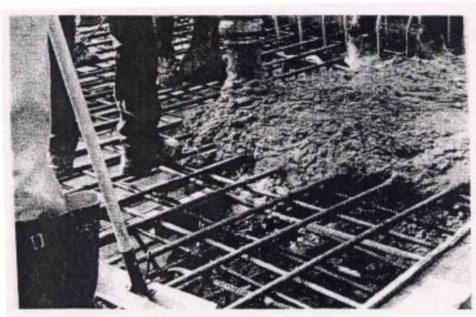
Fig.E.12: Placement of Fresh Concrete at North Main Street Westbound (Connections withstood the construction process)
