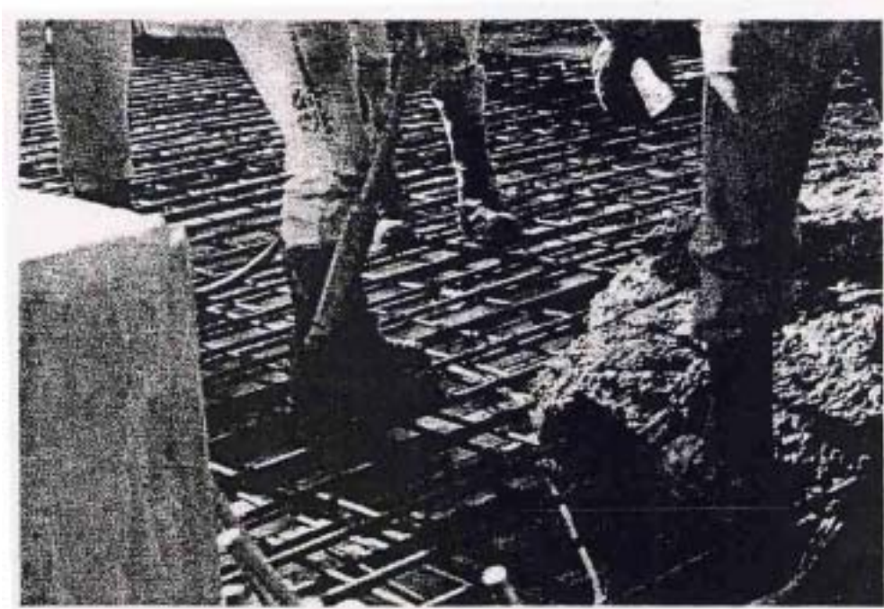
Fig.E.11: Vibrating of Fresh Concrete at North Main Street Eastbound
