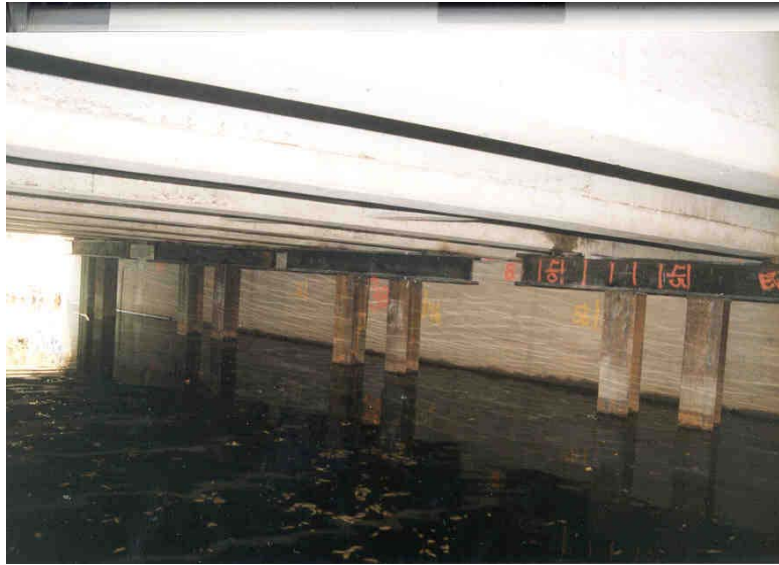
Figure 13.17: Exposed Pile Bents at Peckman's River Bridge on Route 46.
