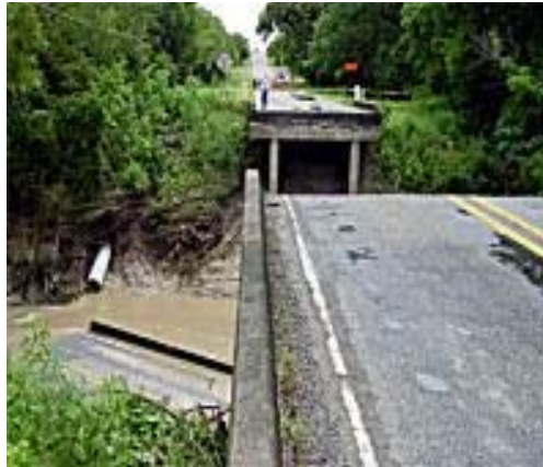
Figure 1.1: Scour Failure of Ovilla Road Bridge in Ellis County, TX on July 20, 2004.
