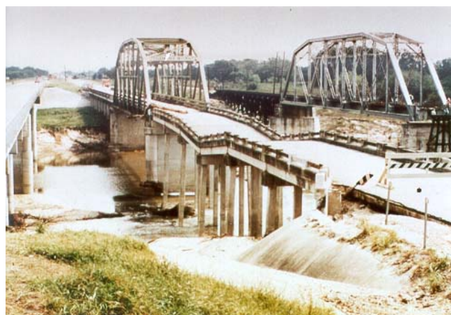
Figure 1.3: Severe damage to a major bridge due to Overtopping of floods.
