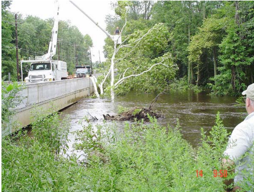
Figure 3.5: Large Floating Debris Accumulation under Lumberton-Vincetown road during July 13-14 2004 flooding
