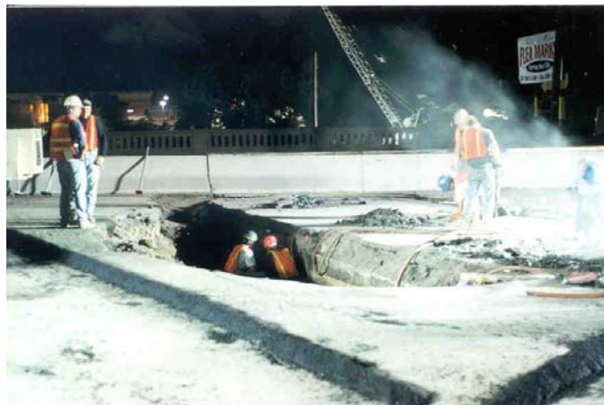
Figure 1.1: Scour Failure of Ovilla Road Bridge in Ellis County, TX on July 20, 2004.
