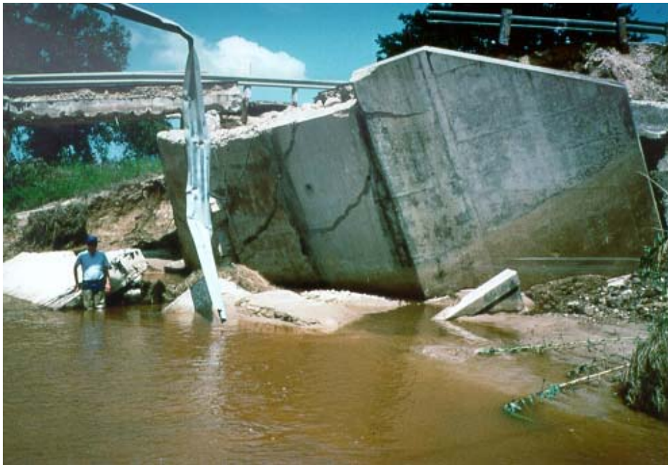
Figure 3.10: Bridge failure due to settlement of foundation in scour hole resulting from deficiencies in foundation design and soil conditions.
