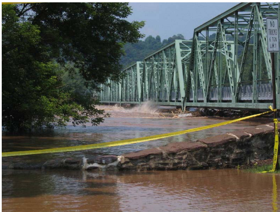
Figure 3.6: Debris accumulation under Frenchtown-Uhlerstown Bridge in Frenchtown, NJ during June 28-30, 2006 flood.
