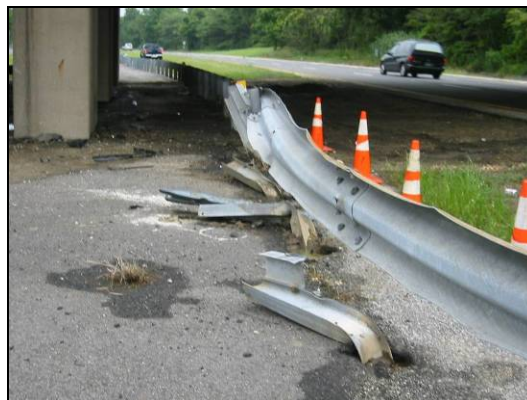
Figure 31. Barrier Damage at I-295 NB MP 25.1
