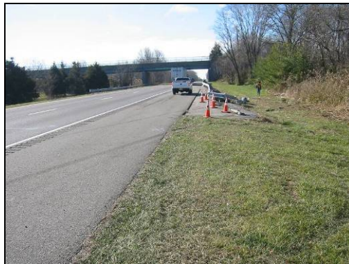
Figure 28. SRT 350 Damage Resulting in Vehicle Rollover and Driver Fatality on I-295 SB
