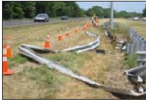
Figure 24. Barrier Damage at I-95 SB MP 6.3
