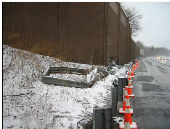
Figure 23. Strong Steel Post Barrier Damage at I-295 NB MP 28.3
