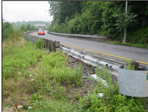
Figure 32. SRT 350 Damage at I-195 WB MP 0.14
