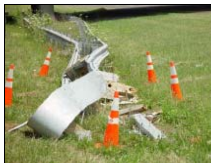
Figure 25. CAT 350 End Terminal Damage at I-95 NB MP 8.1
