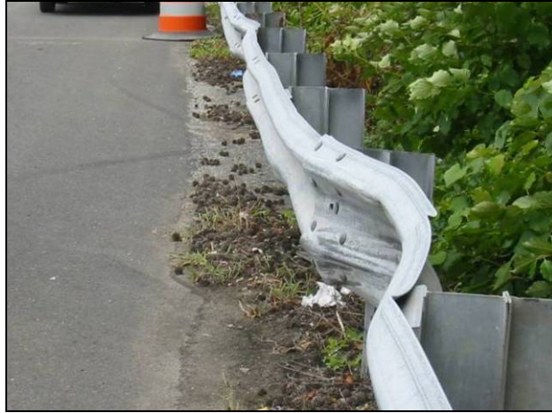
Figure 33. Initial Impact (Foreground) and Second Impact (Background) at State Highway 42 SB MP 12.2
