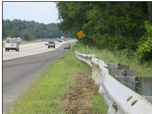
Figure 34. Barrier Damage at I-295 SB MP 43.9
