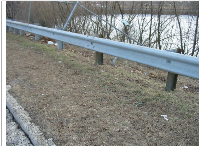
Figure 11. Barrier which contained 1993 Ford Tempo after striking another vehicle.
