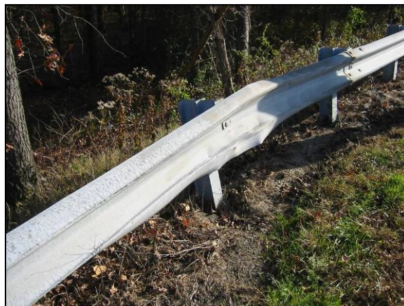
Figure 27. Secondary Impact Damage at I-295 NB MP 64.5
