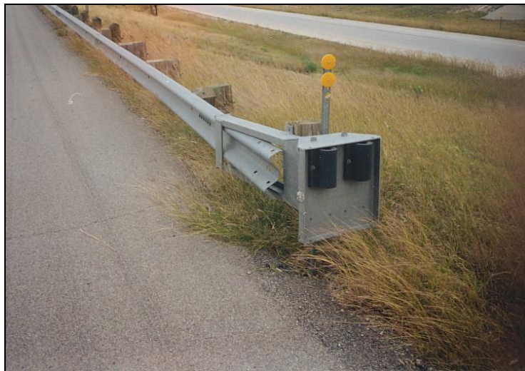
Figure 2. Improper Rail Installation for an Extruder End Terminal
