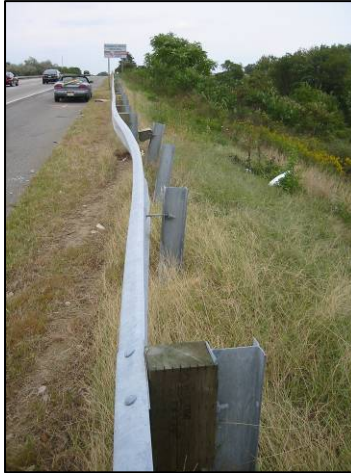
Figure 36. Barrier Damage at I-295 NB MP 41.3
