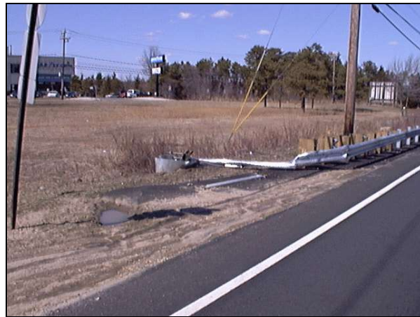
Figure 20. Barrier End Treatment Damage after collision with 1987 Chevrolet Suburban
