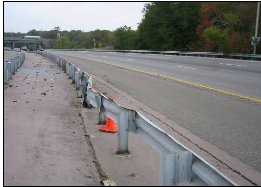
Figure 26. Barrier Damage at I-295 SB MP 14.3
