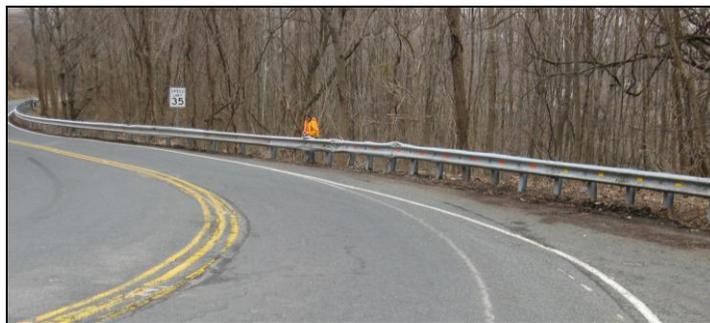
**Figure 45. Damage to guardrail.** There is notable damage to the rail and the posts in multiple areas.
