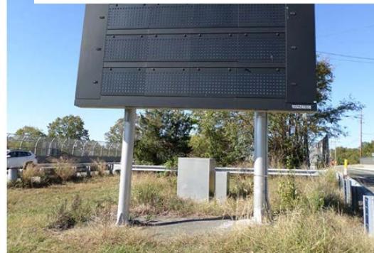
Figure 4. Ground Mounted Structure (Wall, NJ)
