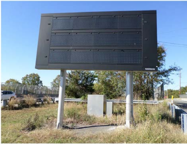
Ground Mounted DMS ID 138 Route 138 WB, MP 2
