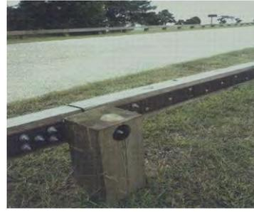
**Steel-backed timber guard rail mounted on wooden posts which has been crash tested and approved by the Federal Highway Administration and has been recently accepted by the NYSDOT for historic parkways**
