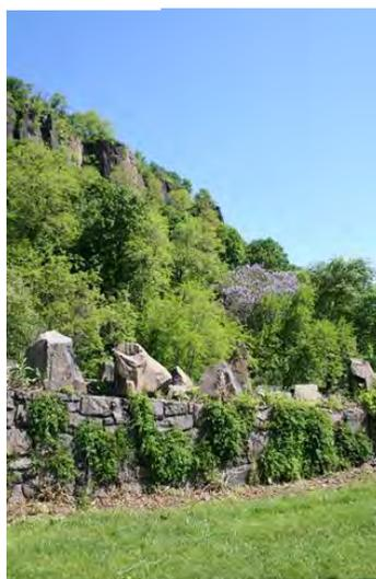
Invasive plant material attached to parapet wall
