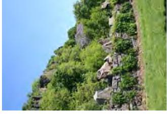
Remove vines and invasive plant material from the parapet walls. Vines will weaken the wall structure and should be removed as part of a continuous maintenance program throughout the year.
