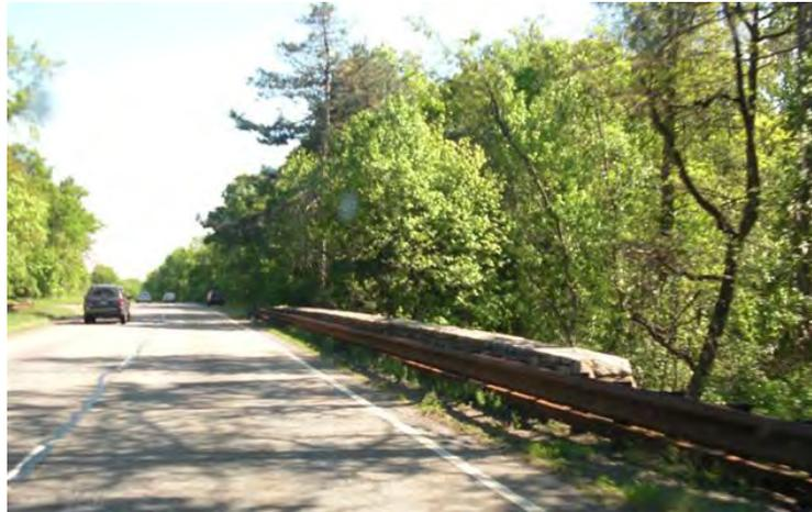
**Existing photo of the metal guardrails in front of the original bridge rails on the New Jersey section of the Palisades Interstate Parkway**
