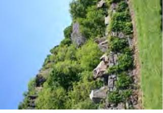
Remove vines and invasive plant material from the parapet walls. Vines will weaken the wall structure and should be removed as part of a continuous maintenance program throughout the year.
