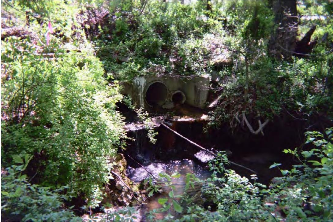
Photo Plate 39: View of inlet pipes conveying flow (Waters of the U.S. in Culvert) under Bellmawr Park. Note severe scouring of stream bank and structure.
