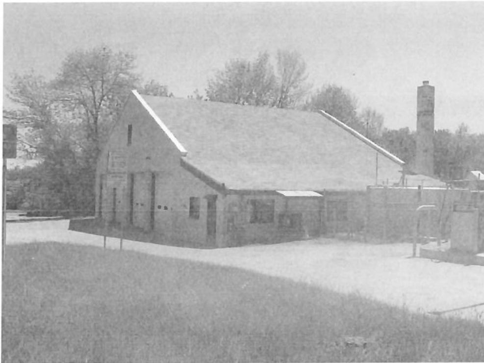
LBAM Building ID: 1209 Office & Garage (Front View)
