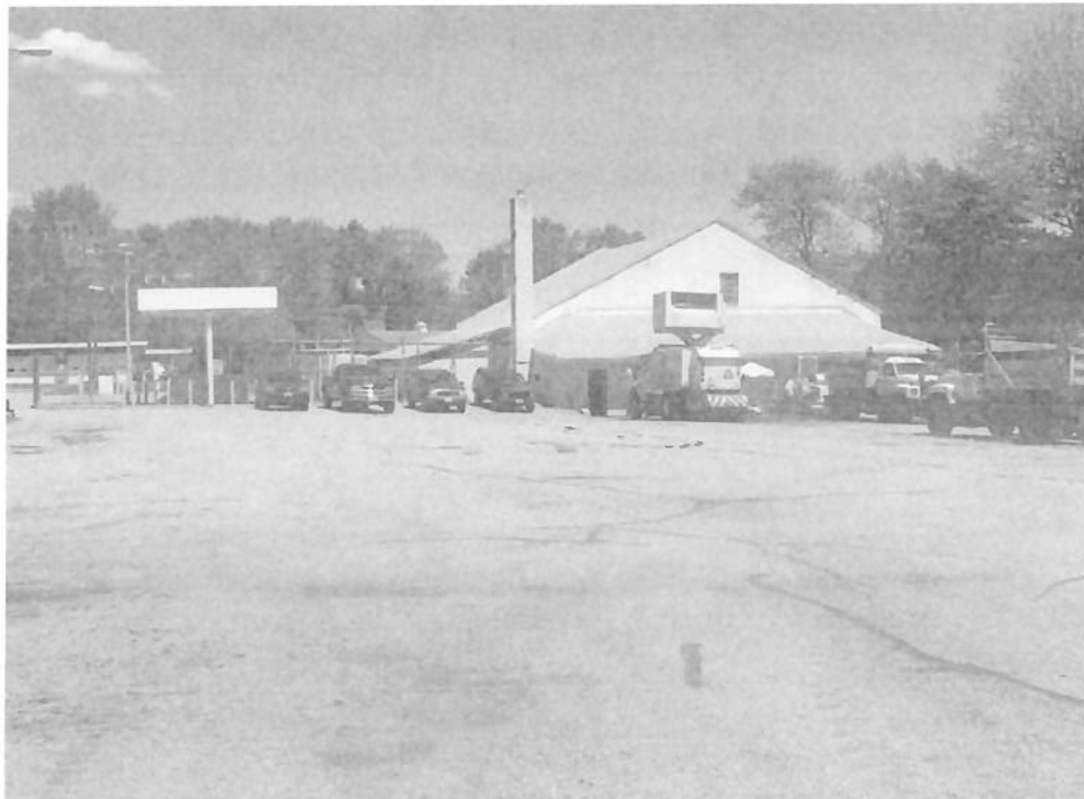
LBAM Building ID: 1209 Office & Garage (Rear View)
