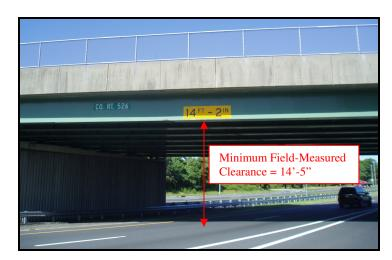
C. <u>Unacceptable</u> because safety factor is <u>less than</u> 3 inches (inspector must write PR-1 Memo to correct).
