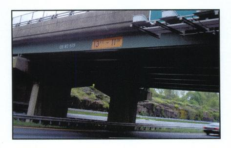
Case B. Each travel lane has its own posting sign indicating the minimum vertical clearance for that particular lane
