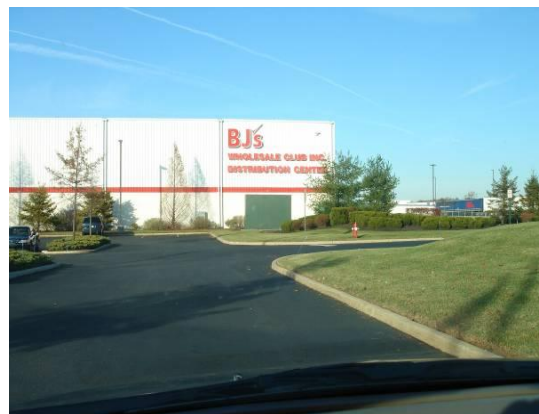
BJ’s Wholesale Club Distribution Center at the Haines Industrial Center
