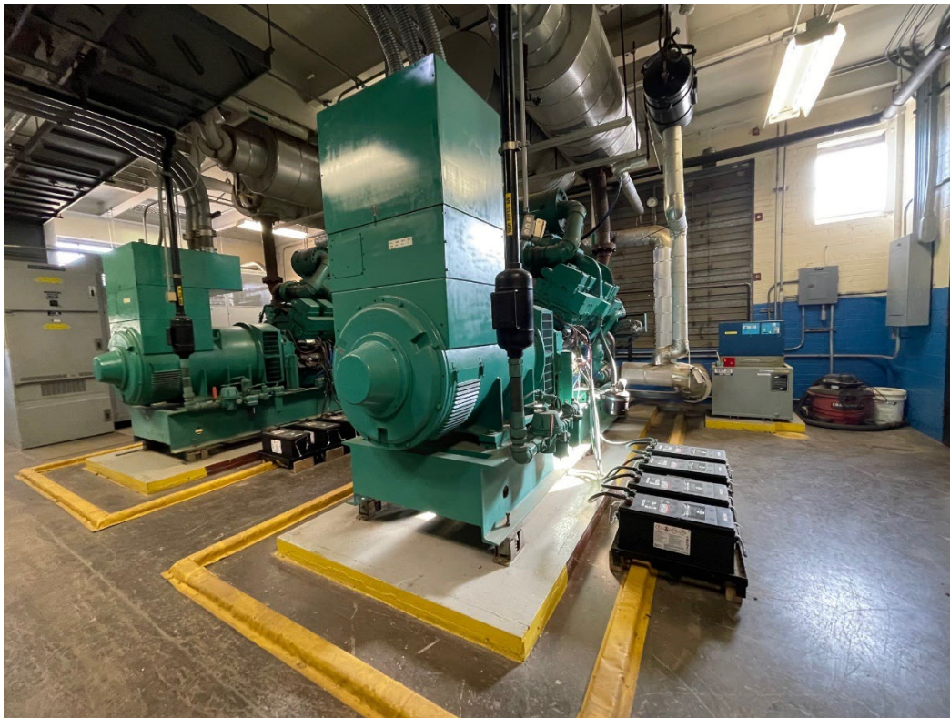
750 KW Generators to be replaced.
