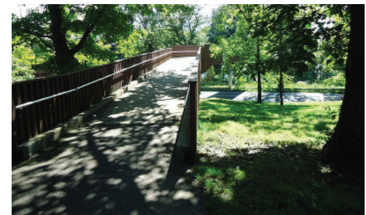
Photograph 8. Pedestrian footbridge over New Jersey Route 29, which was constructed in 1976
