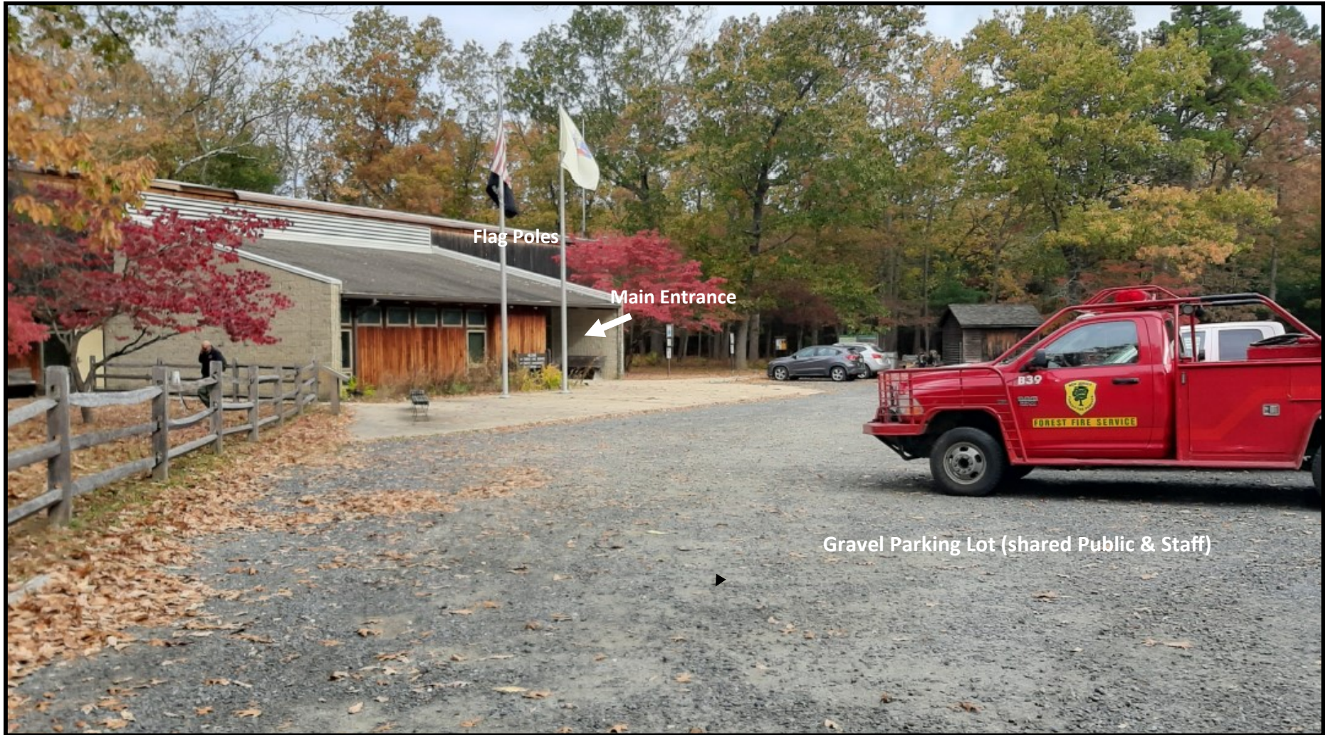
Office Building - front view
