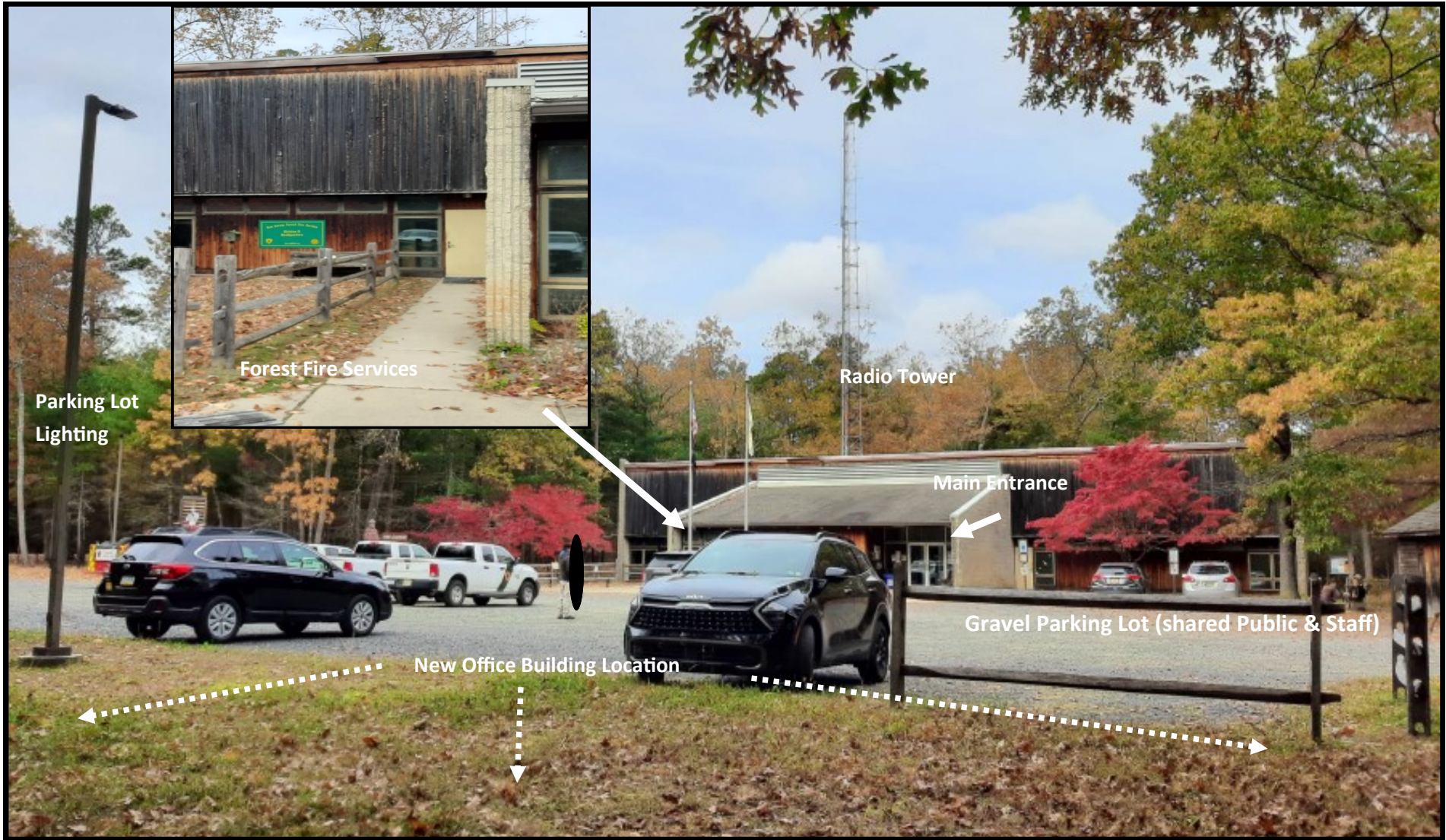
Office Building - front view
