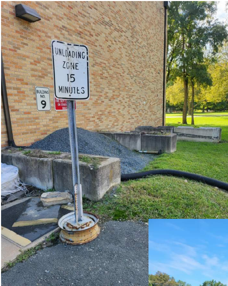
Existing Exterior Material Storage Bins for Aggregates
