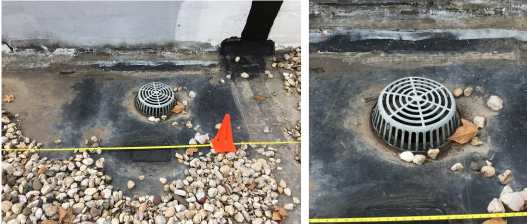
Drain at leak area along south parapet – torn membrane at SW side of drain body
