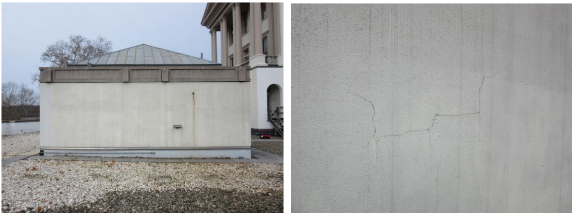
Cracked Stucco at East Wall of Mechanical Penthouse
