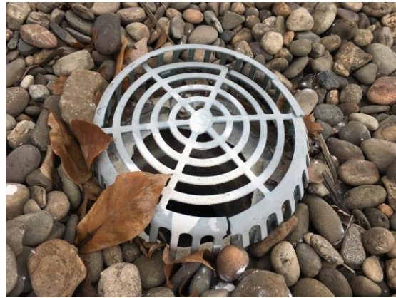
Debris at drain / broken dome
