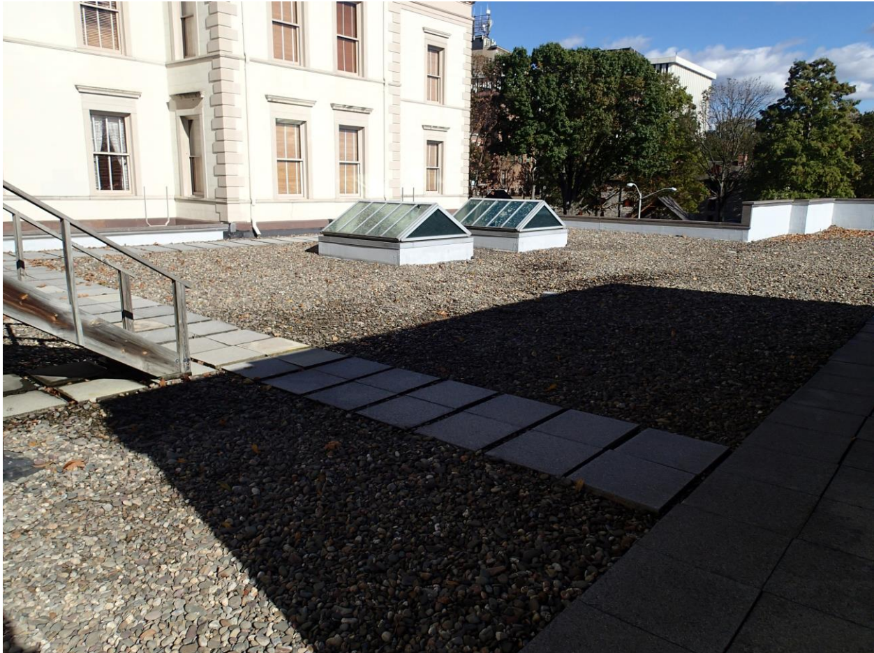
LSH Low Roof (East Side) – Ballasted EPDM
