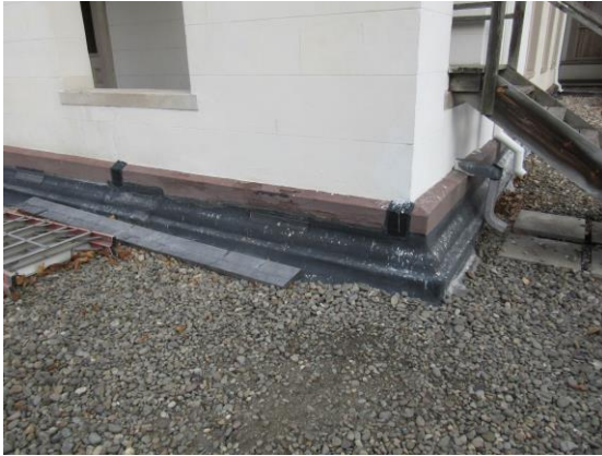
Dirt/Debris left in ballast at Portico/Steps
