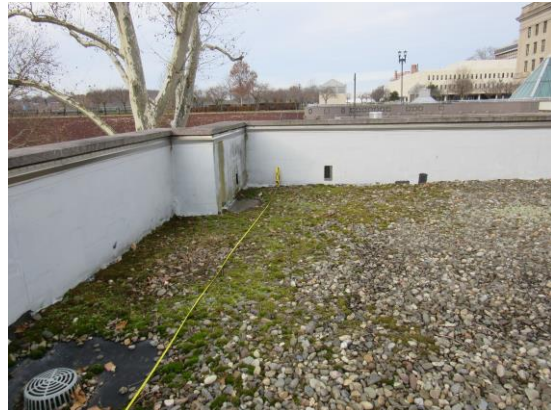
Organic debris in ballast at SW corner
