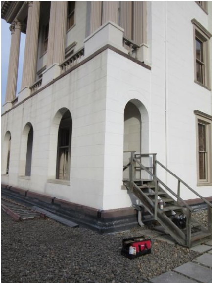
Area of leak when roof was flooded during pressure washing activities
