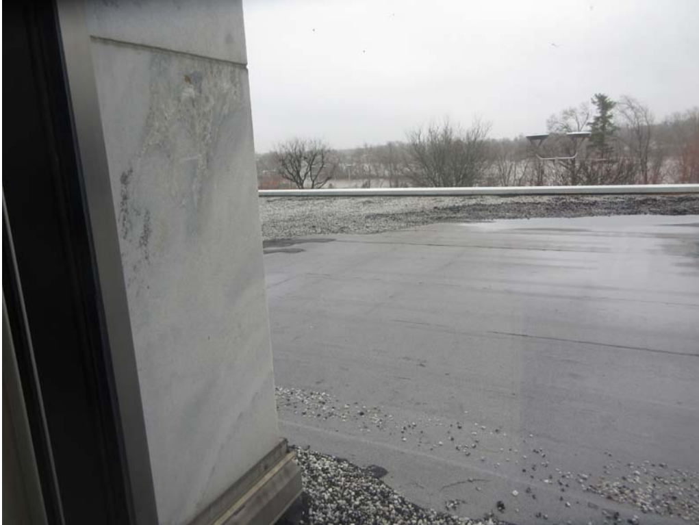
3. Roof Area C: Additional view at the repaired area.
