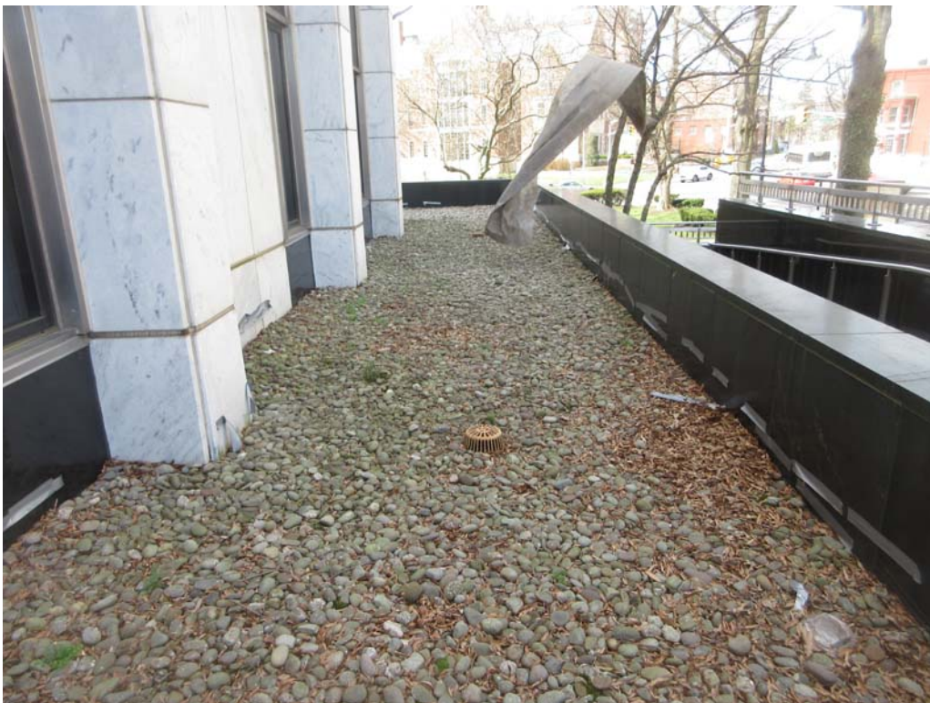
1. Roof Area E: Partial overall view looking southwest on Area E showing numerous repairs made with duct-tape on the wall panels.
