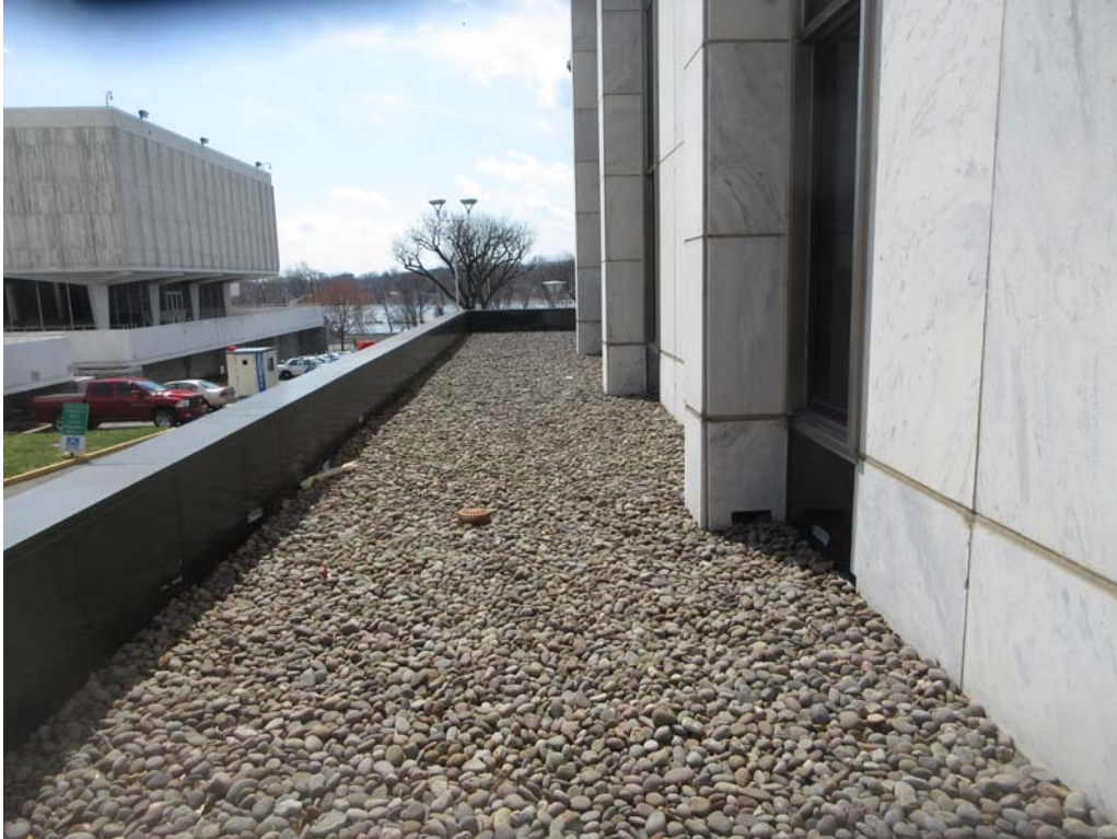
4. Roof Area D: Additional partial overall view.
