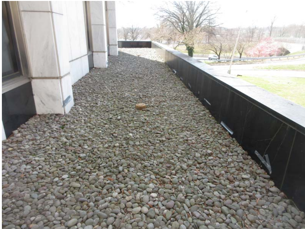
3. Roof Area E: Additional view of Area E.
