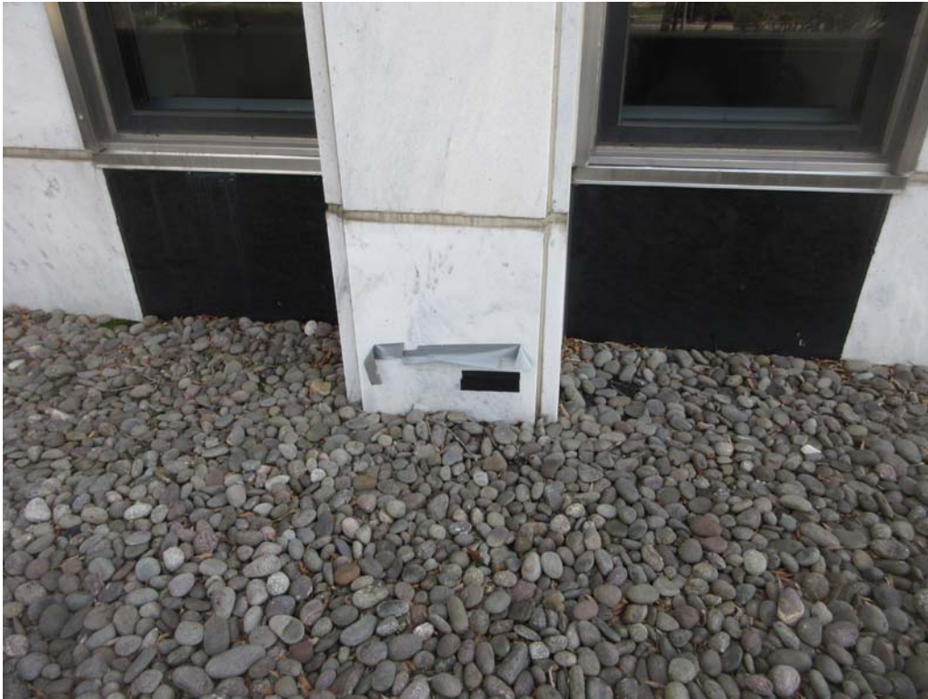
4. Roof Area E: Close-up view of the marble wall panel on Area E.
