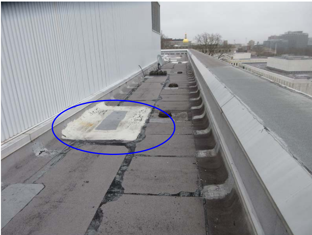
14. Roof Area B: Recent repairs made on Area B (whiter materials).
