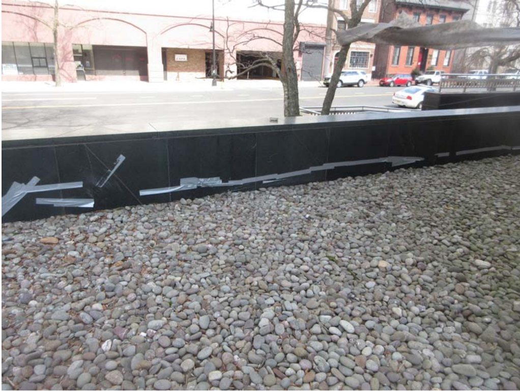
2. Roof Area E: Another partial view of Area E; here again, duct-tape was used to cover splits in marble wall panels.
