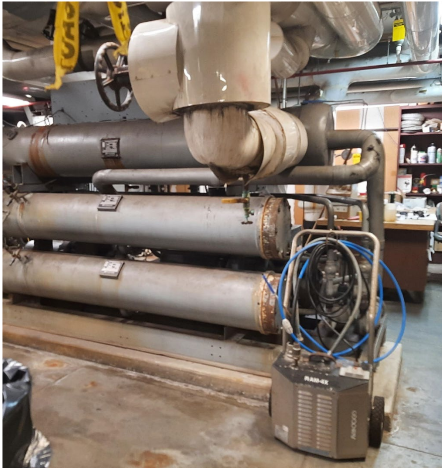
Chiller equipment at Building 74 to be disconnected.
