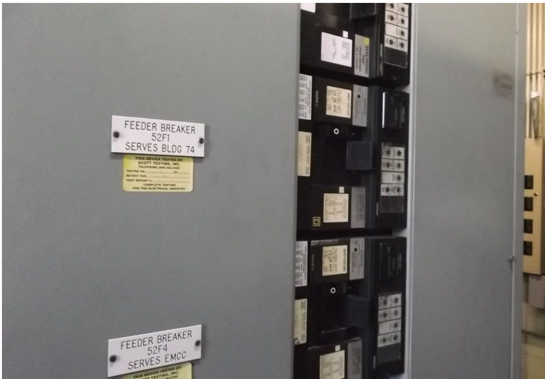
Electrical equipment in Lab from which electricity is fed to Building 74.
