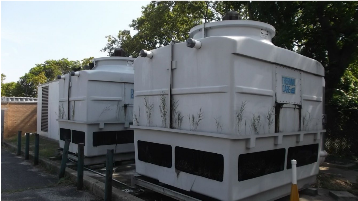
Cooling Towers at Lab from which chilled water is supplied to Building 74.
