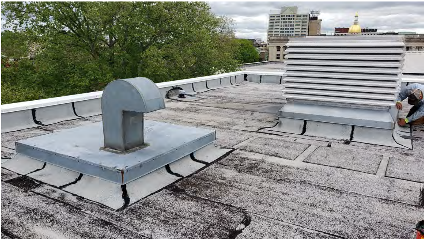
Rooftop Vents at Penthouse Roof
