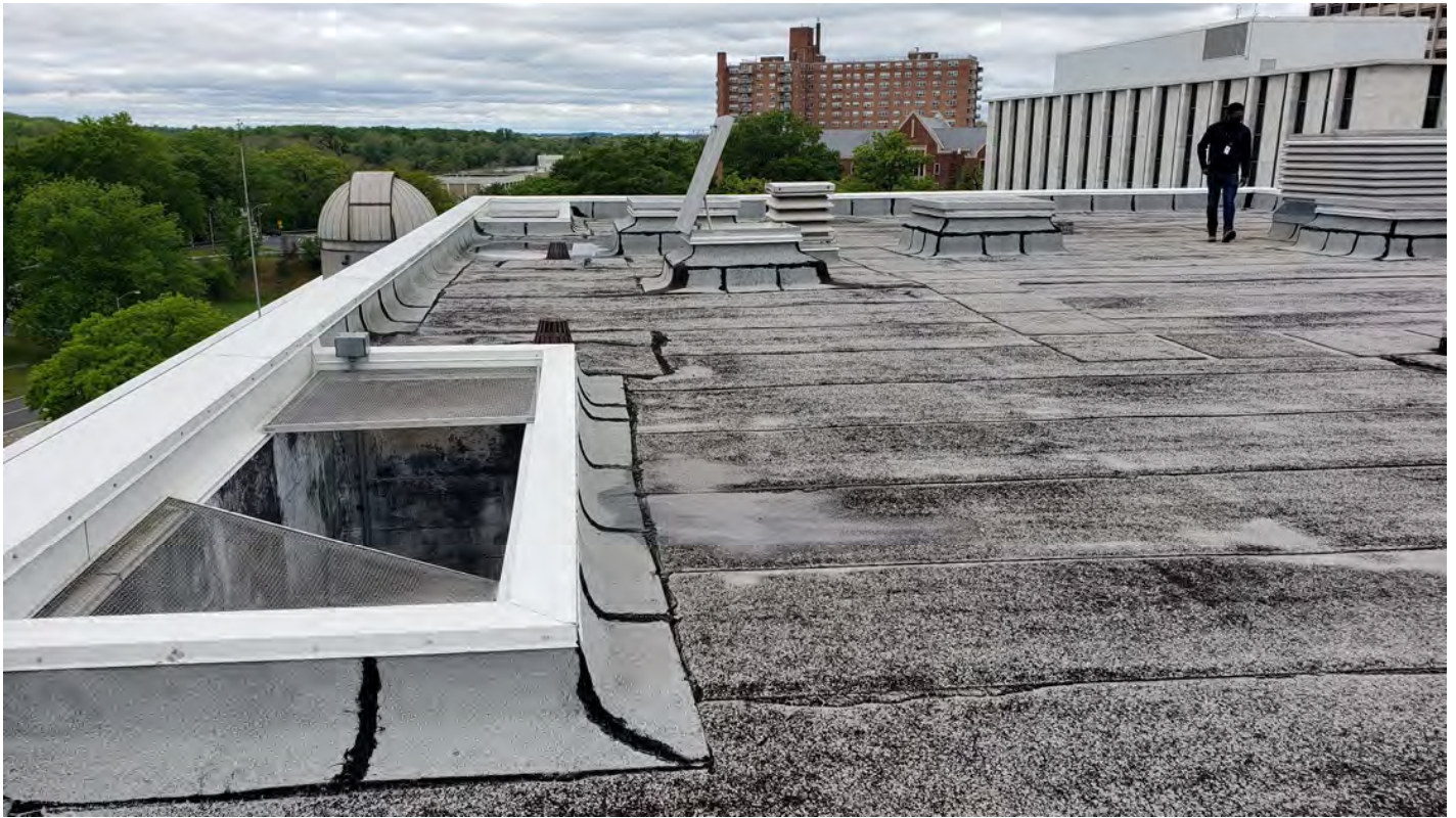
Penthouse Roof Looking West
