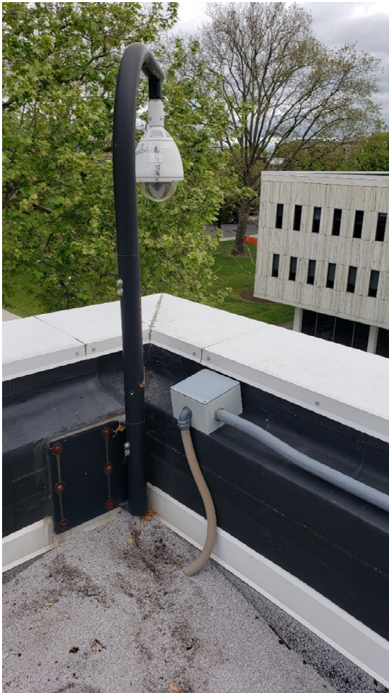
Existing Camera, Coping, Junction Box, and Conduit at Northeast Corner of Main Roof. Note Build-up of Dislodged Cap Sheet Granules and Inner Shelf at Parapet Wall Covered with EPDM Membrane
