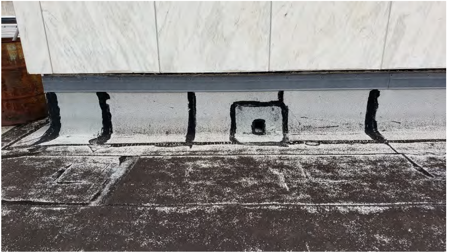
Drainage Outlet at Base of Air Shaft
