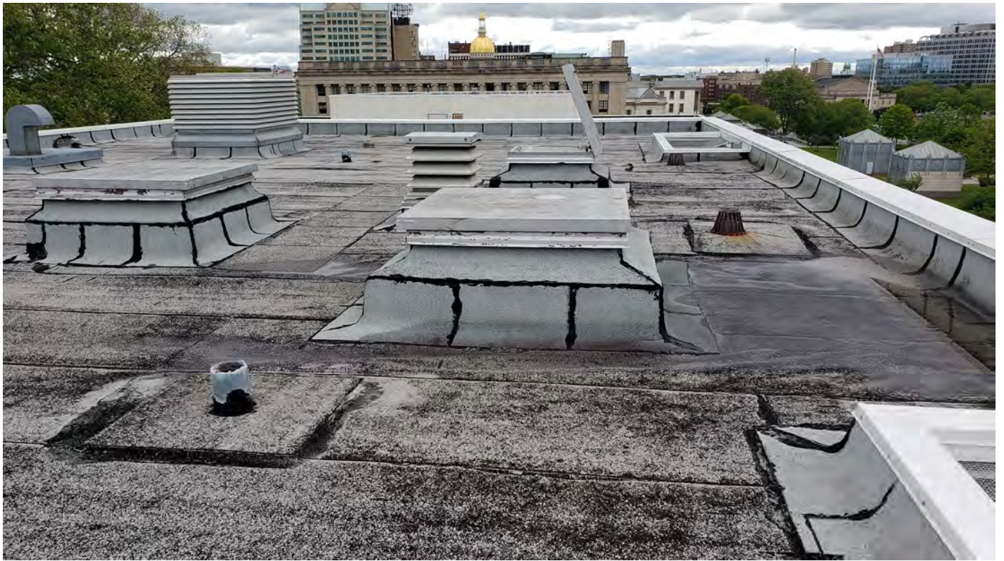
Penthouse Roof Looking East
