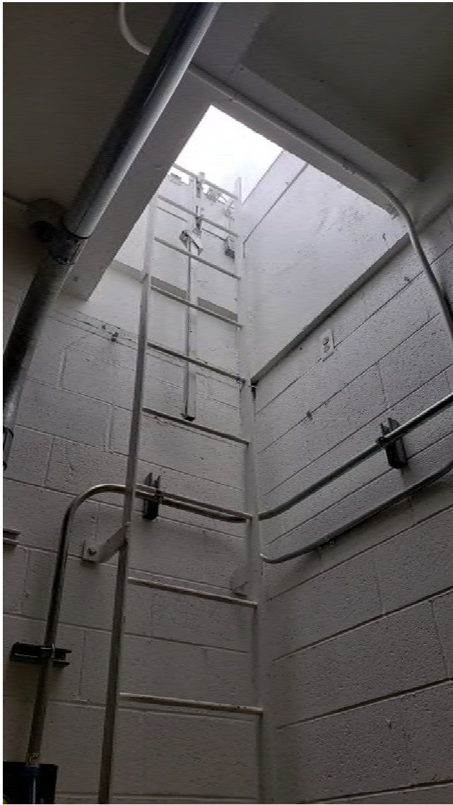
Roof Hatch Opening to Penthouse Roof
