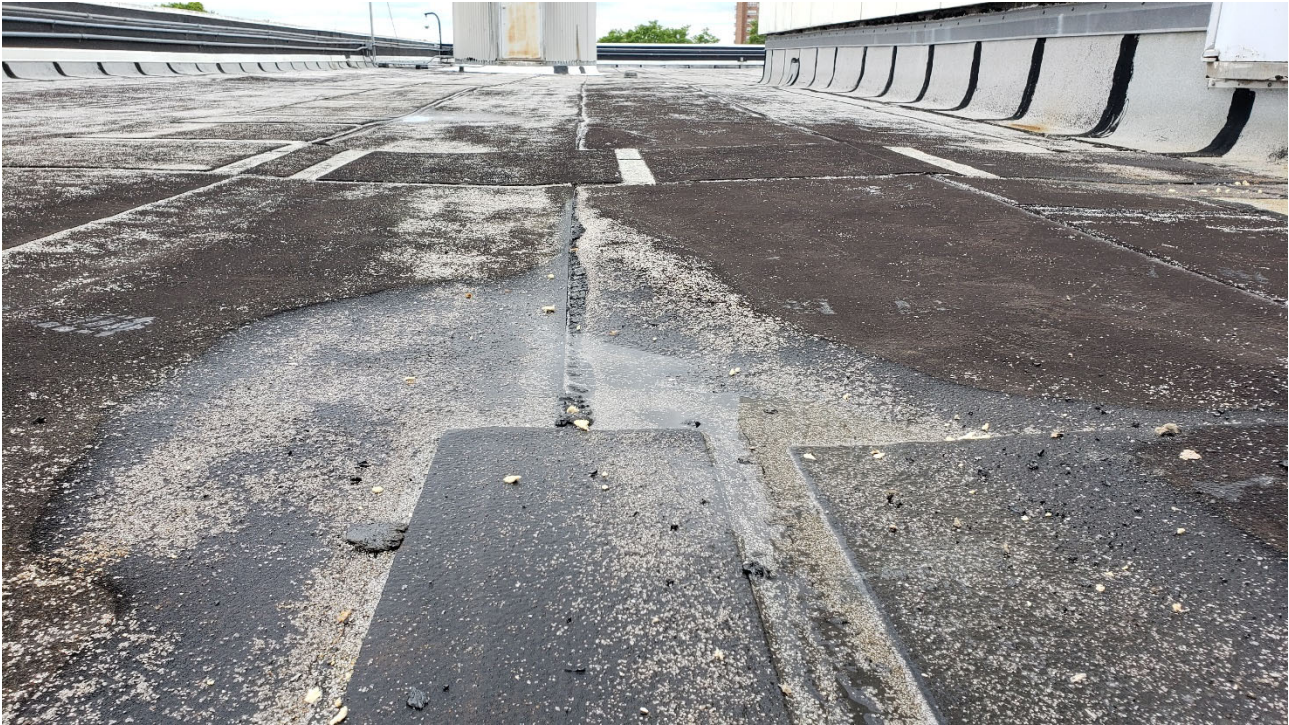
Main Roof South Side.
