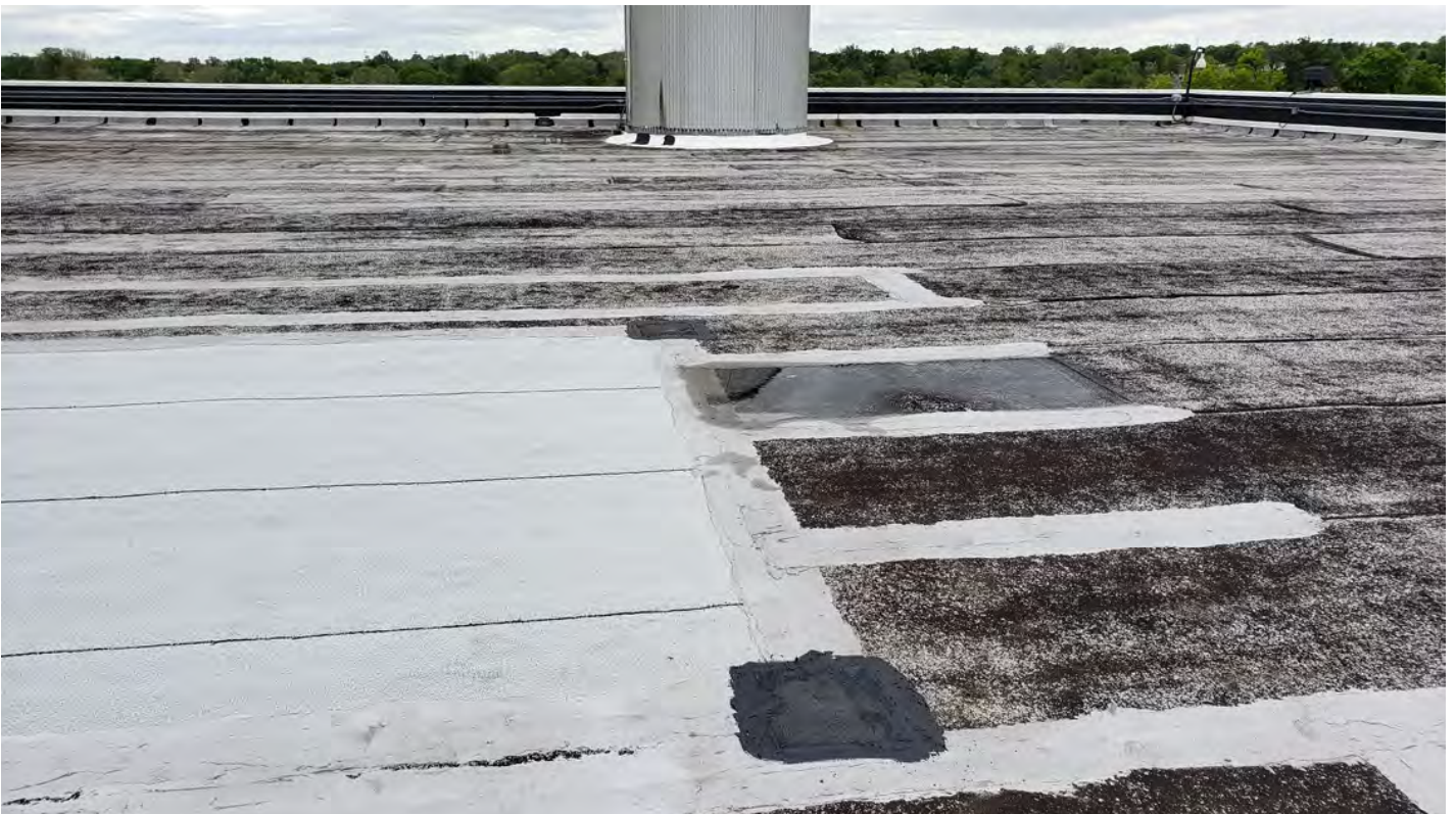
Field of Main Roof, West Side, at Previous Patch
