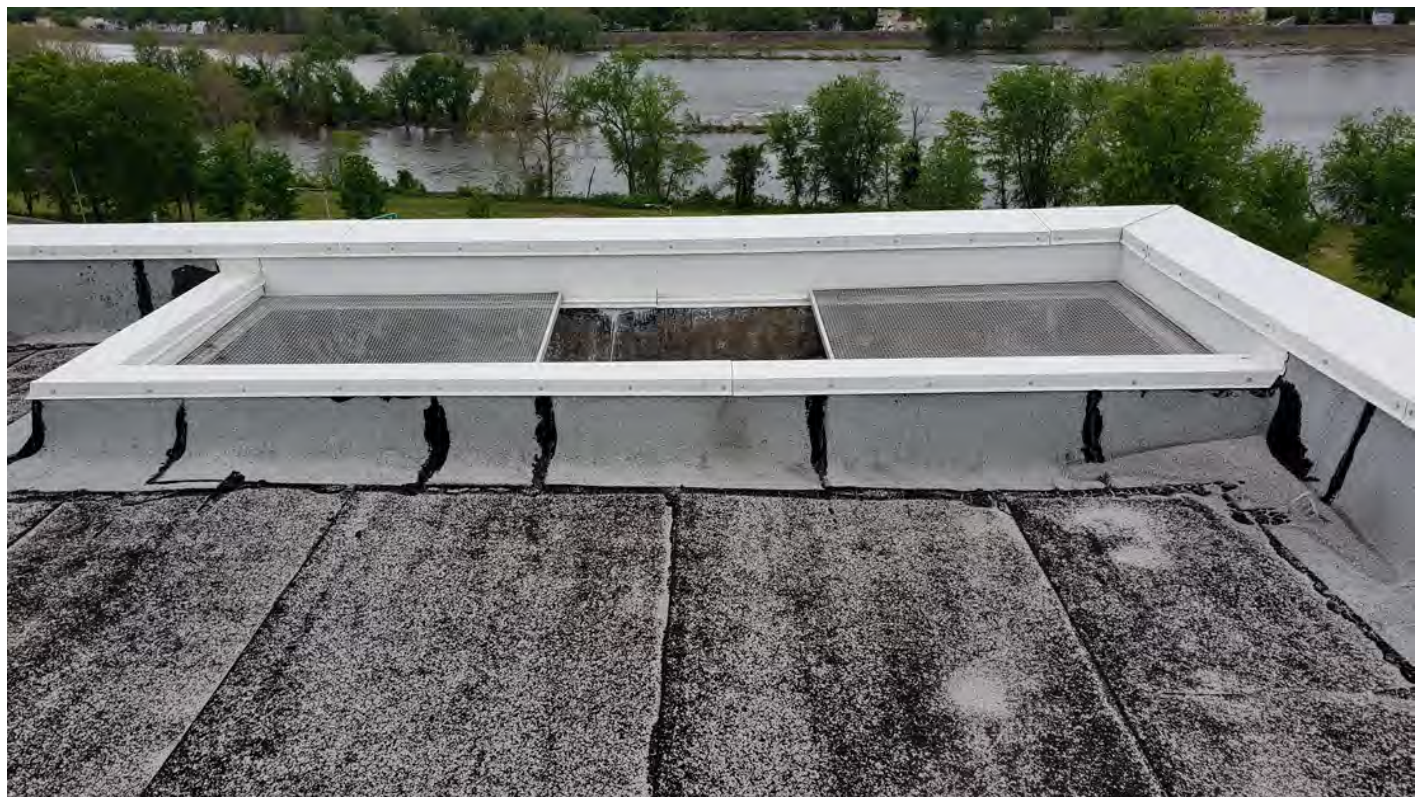
Top of Air Shaft at Penthouse Roof
