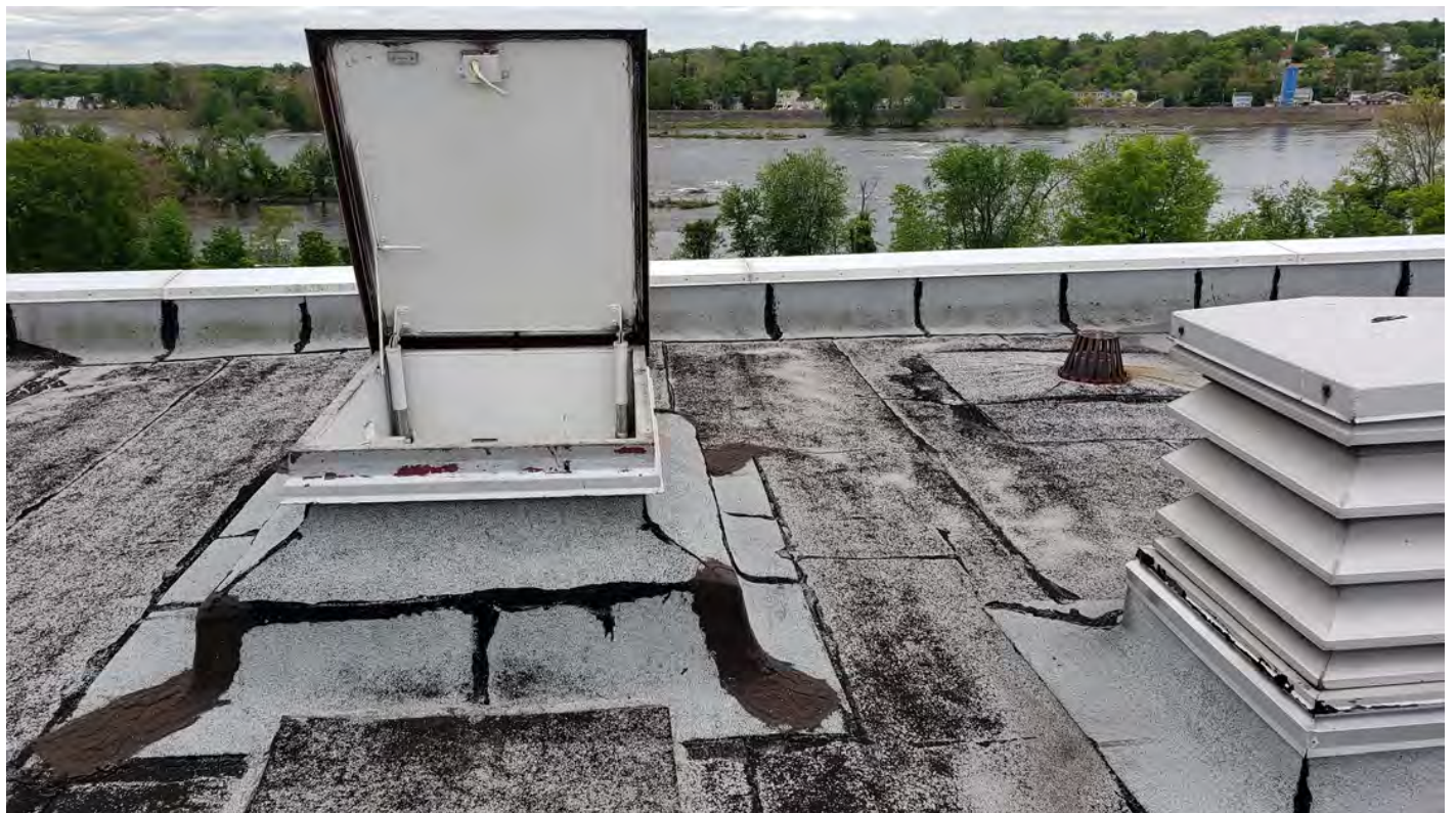
Roof Hatch at Penthouse Roof
