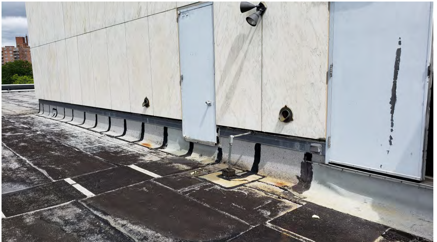
Conduits Down Though Pitch Pocket Into Roof Insulation. Drainage Outlets From Penthouse Overflow Drains
