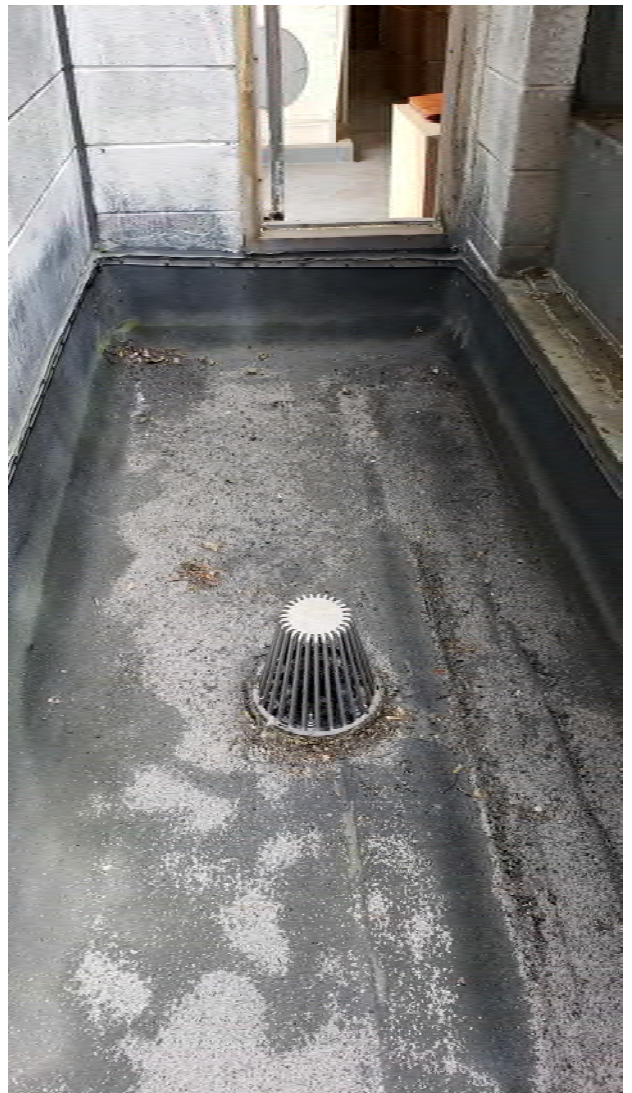
EPDM Roof at Base of Air Shaft
