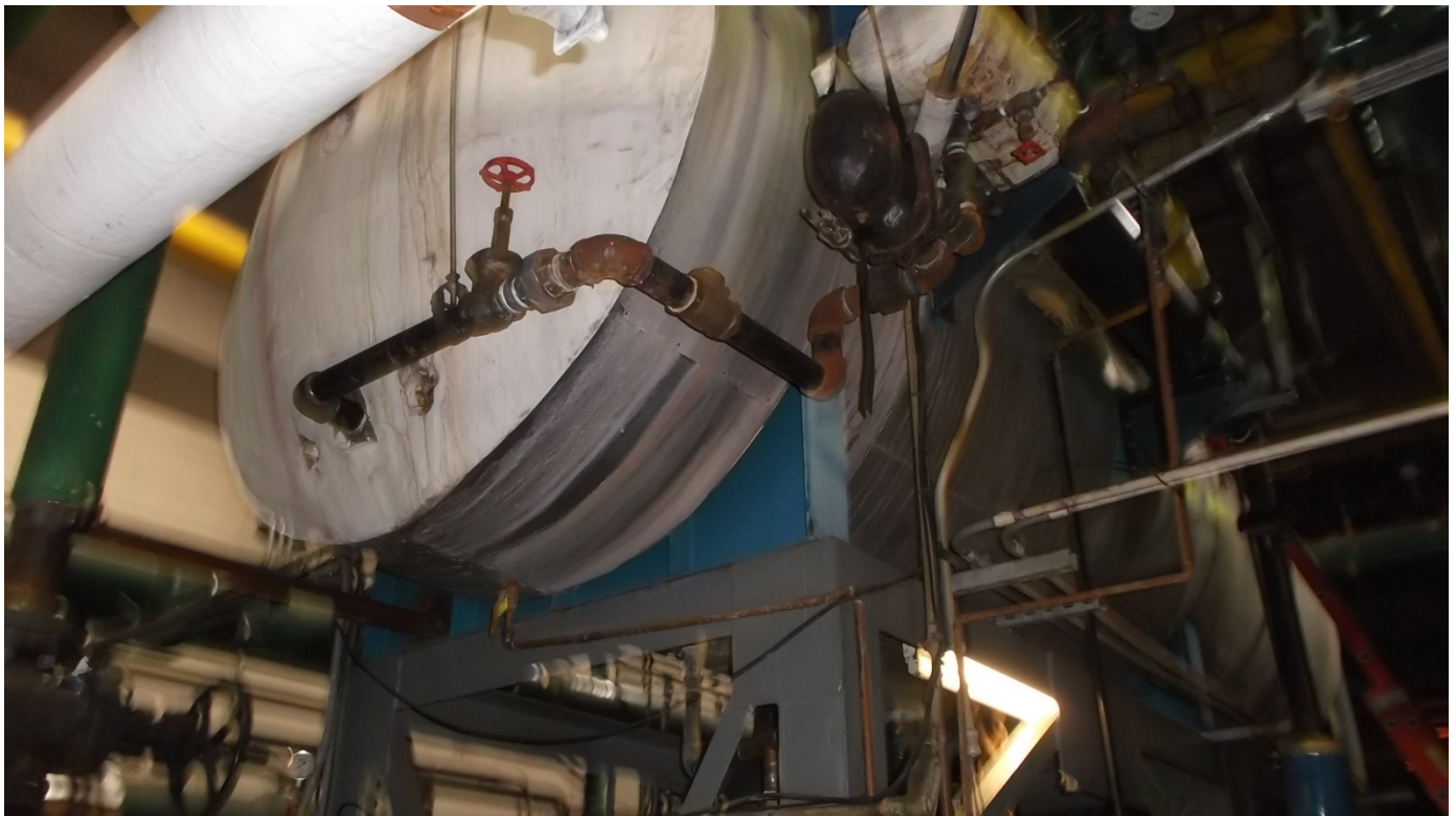
Deaerator Tank in Powerhouse at Trenton State Prison. EXHIBIT 'D'
