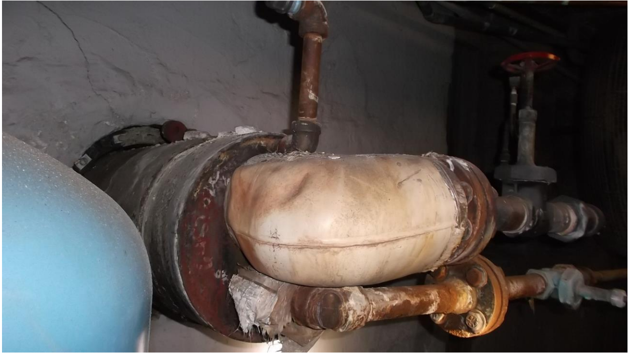
Steam Condensate Supply & Return Pipes and Valves in Basement Of Wing 6, to be replaced.
