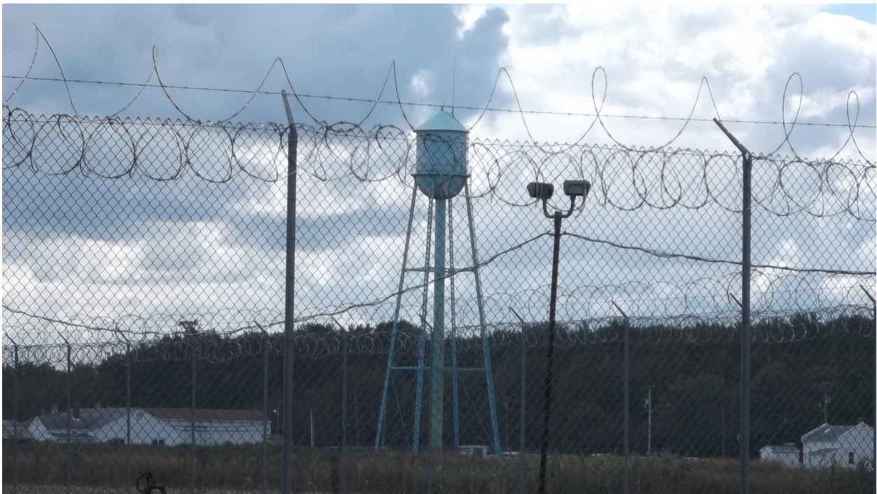
Bayside State Farm & Dairy-Water Tower #2- Storage Capacity of 80,000 gallons
