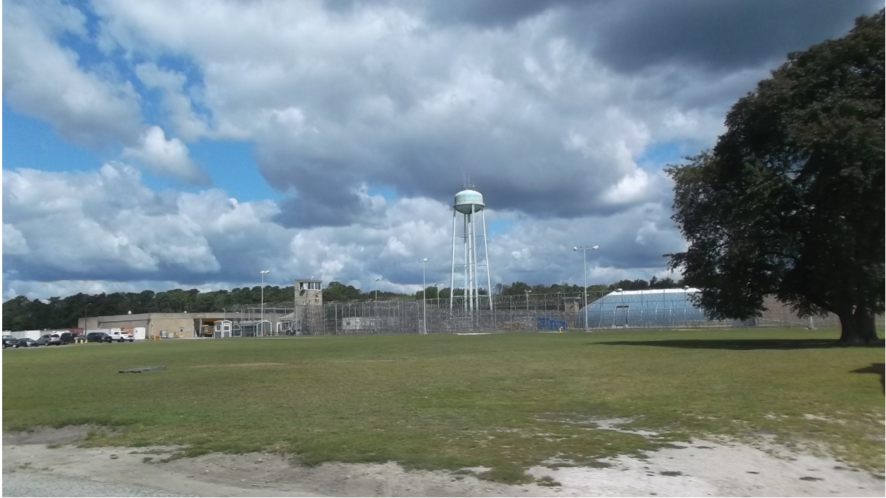
BSP Water Tower #1- Storage Capacity of 100,000 gallons
