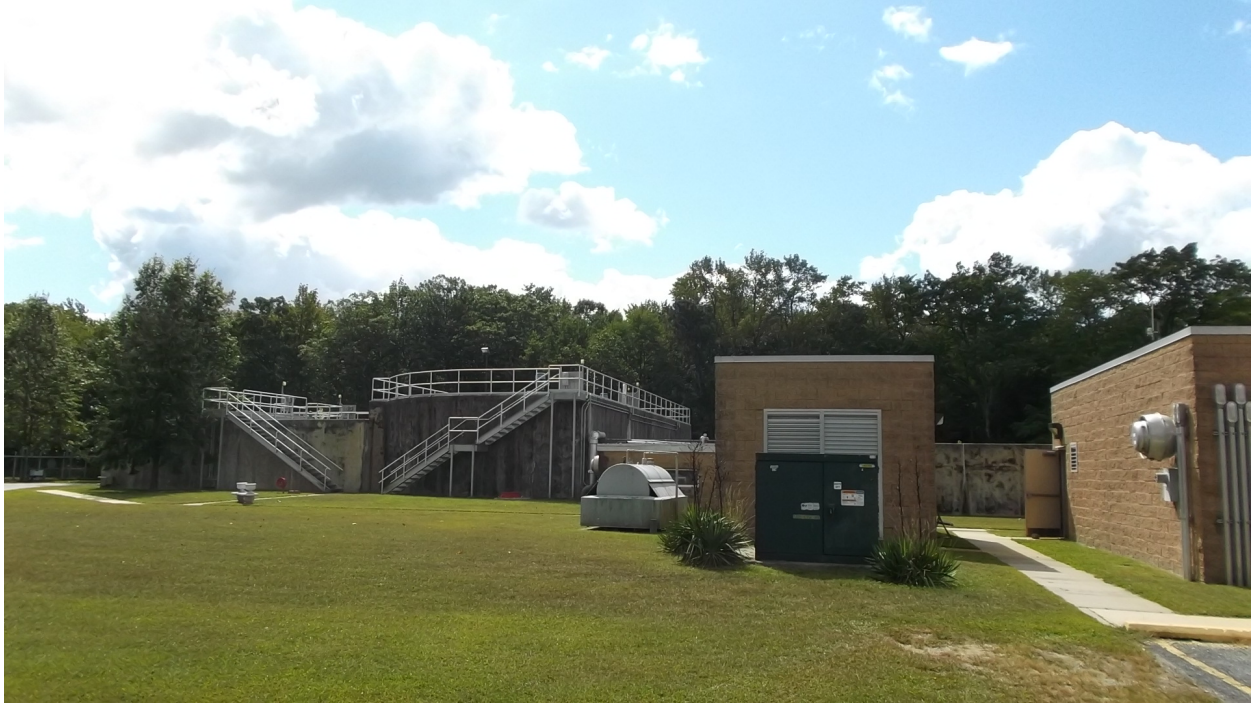
Bayside State Prison Sewer Plant
