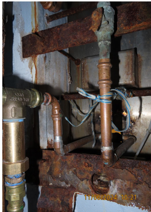
Figure 4 Shower control panel support brackets
