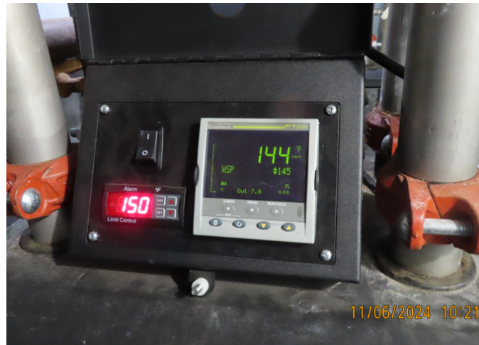
Figure 1: Aerco heater temperature settings
