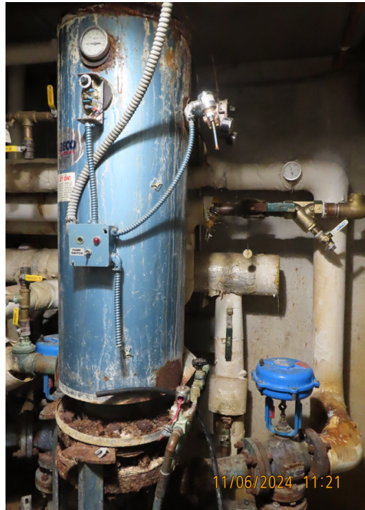
Figure 5 ACSU 1&2 Domestic Hot Water Heater
