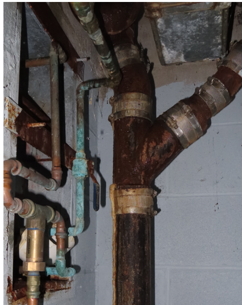
Figure 2: Active leak at waste stack
