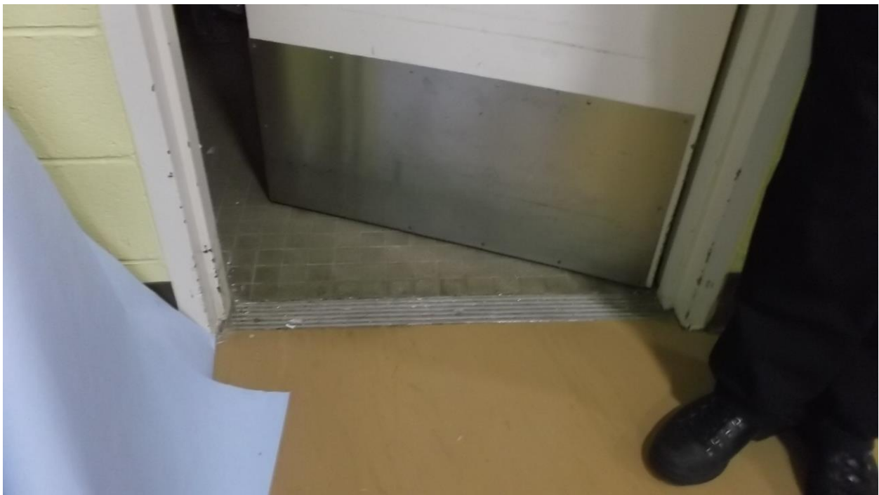
Gymnasium Flooring along the Entry to tiled Adjacent Spaces
