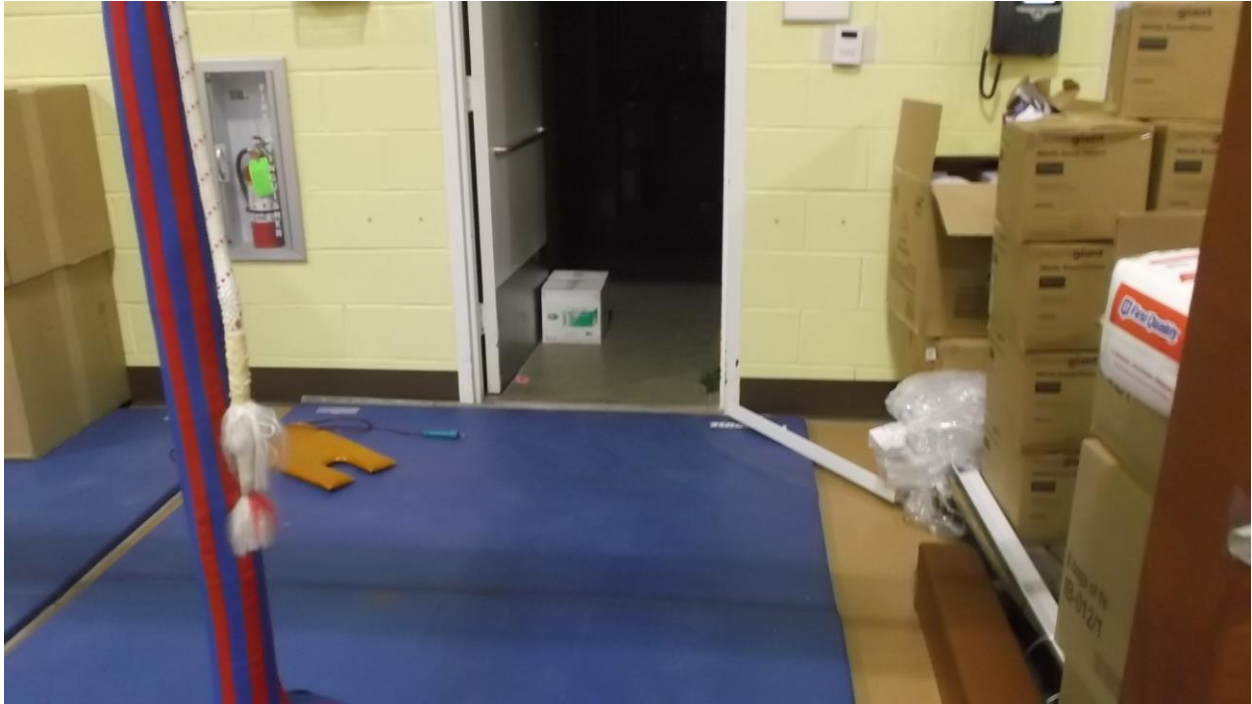
Gymnasium Flooring along the Entry to Adjacent Spaces.
