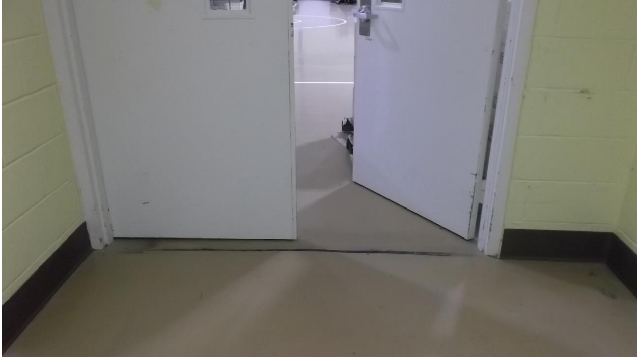
Gymnasium Entry To Connecting Hallway
