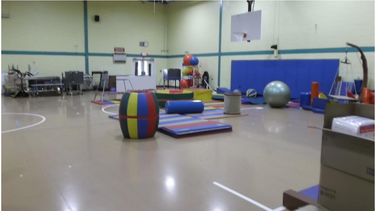
Gymnasium Rubber Floor to be replaced
