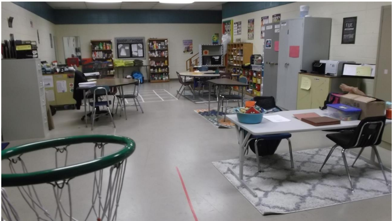
PT/OT Classroom Floor to be replaced
