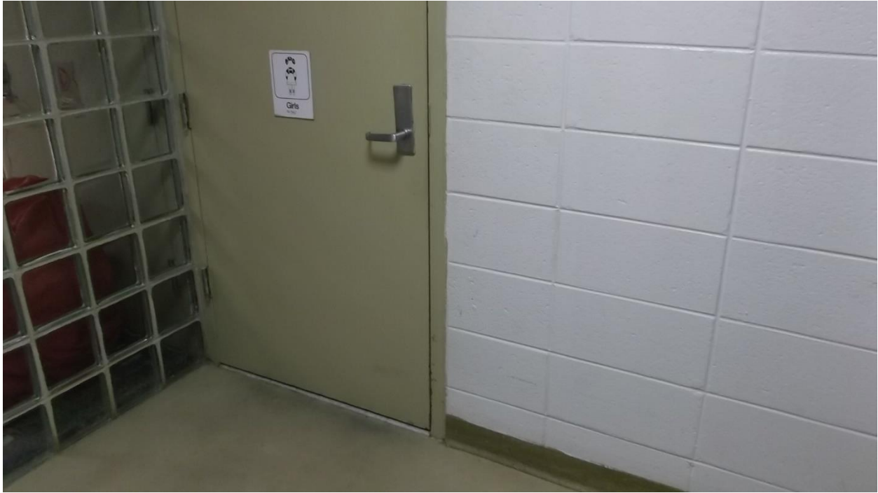
Connecting Hallway between Gymnasium and OT/PT Classroom
