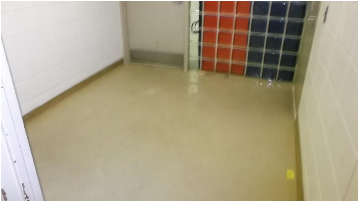
Connecting Hallway between Gymnasium and OT/PT Classroom
