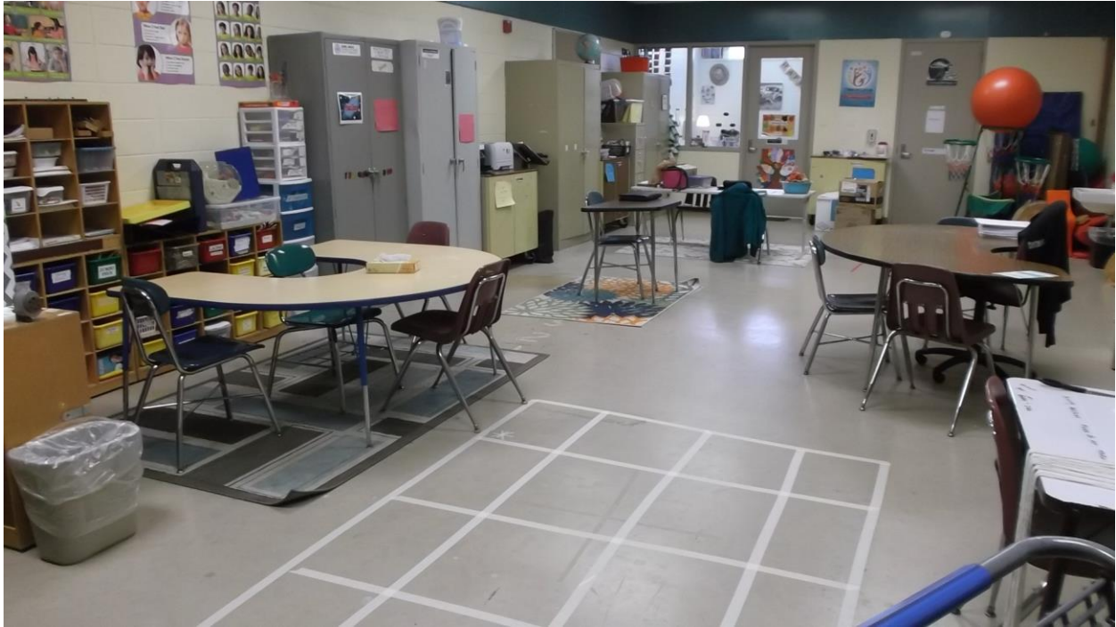
PT/OT Classroom Floor to be replaced
