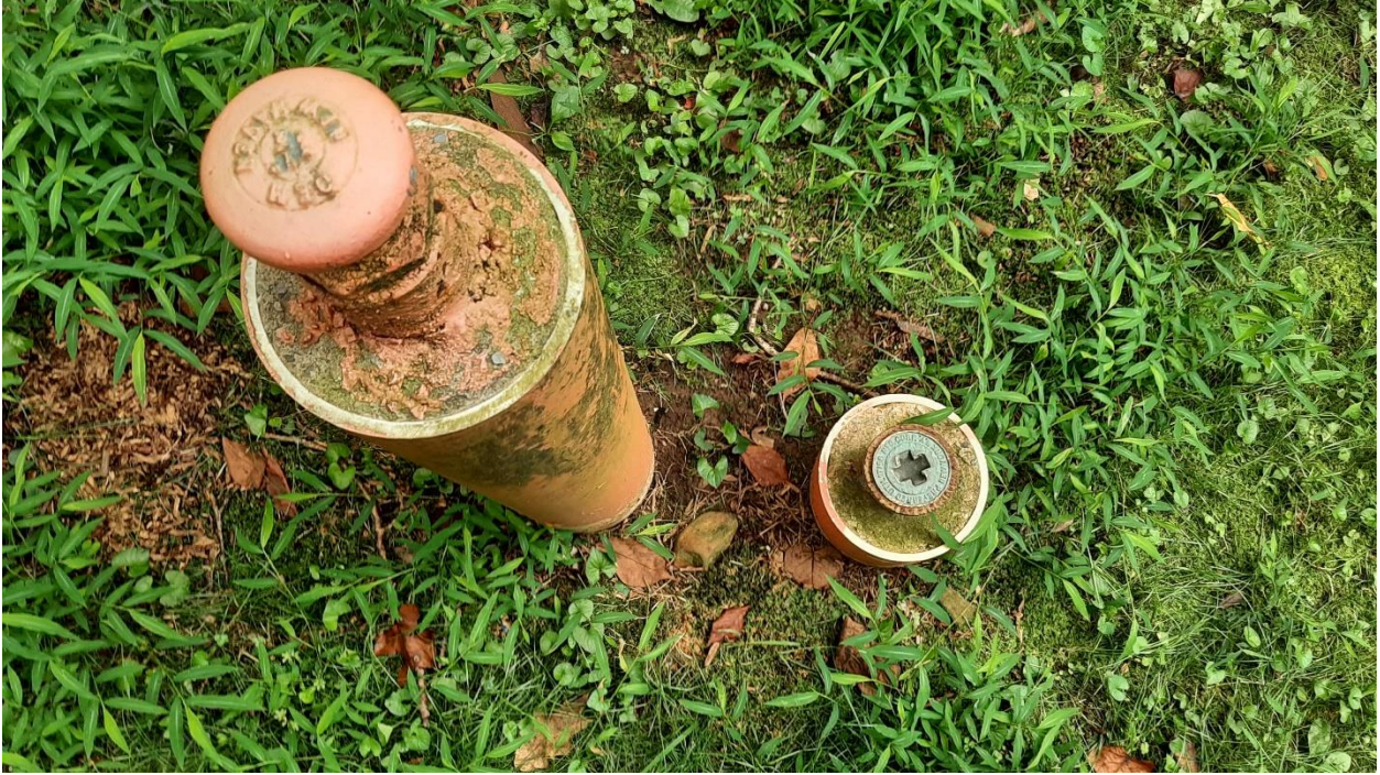
Existing Underground Diesel Fuel Storage Tank to be removed.
