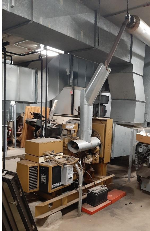
Existing Building Diesel Powered Generator to be replaced.
