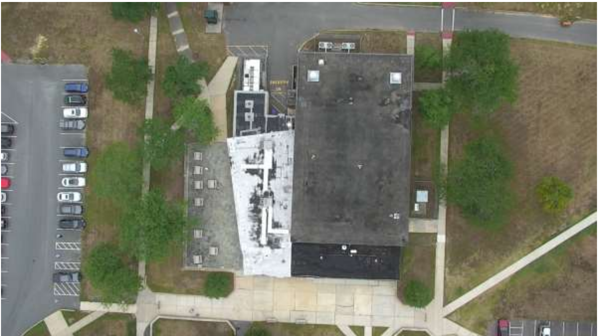
Existing Roof Conditions of The Ivy Hall and Anorage .
