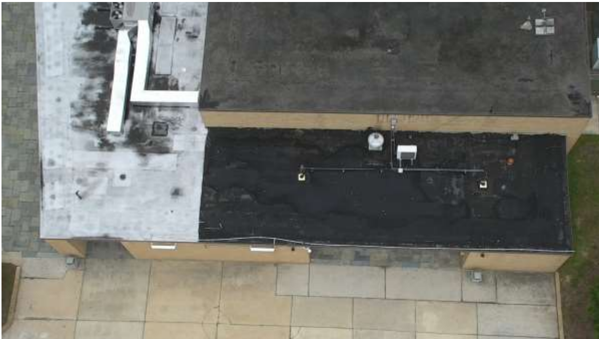
Existing partial lower level – Anchorage Roof.
