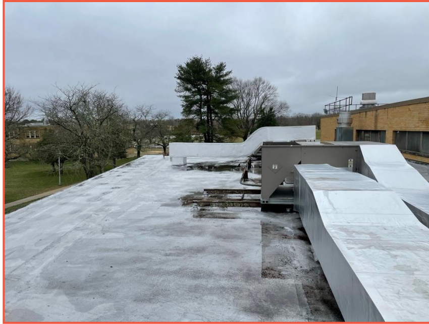
Photo No 1. Top of Ancorage Roof
