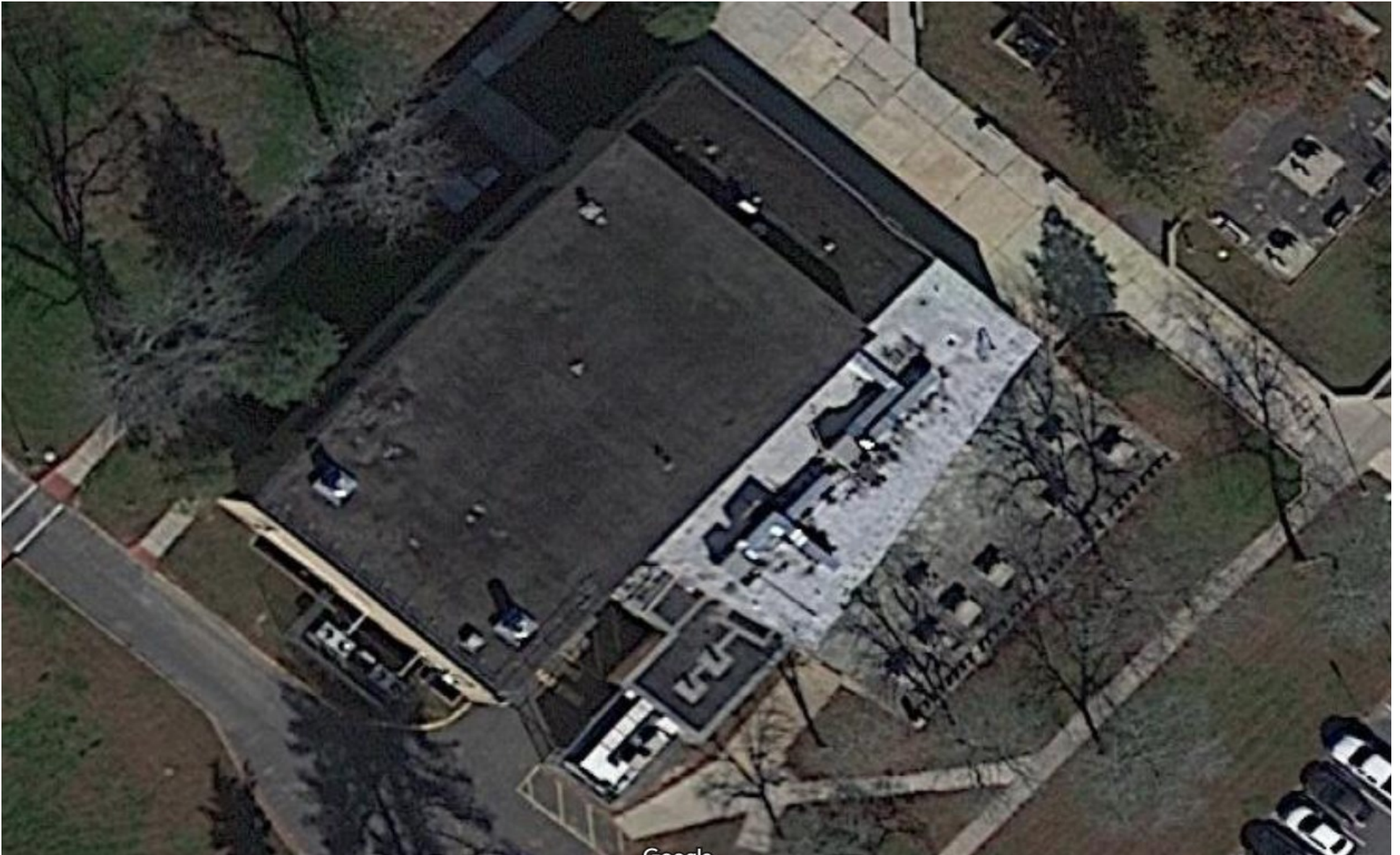
Ivy/Ancorage Roof Aerial view
