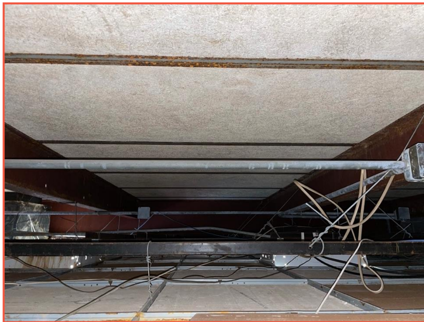
Photo No 3. Ancorage Roof Underside
