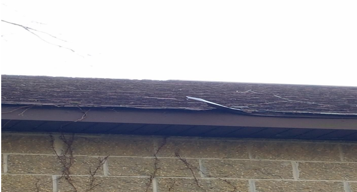
Existing conditions of failing roof shingles and failing gutters.
