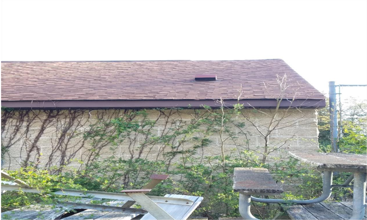
Existing missing Ridge Vent
