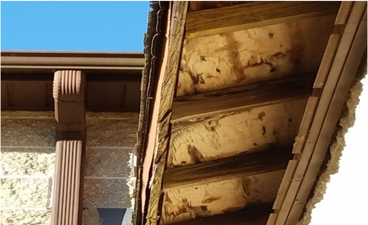
Missing soffit, gutters deteriorated fascia and water damage.
