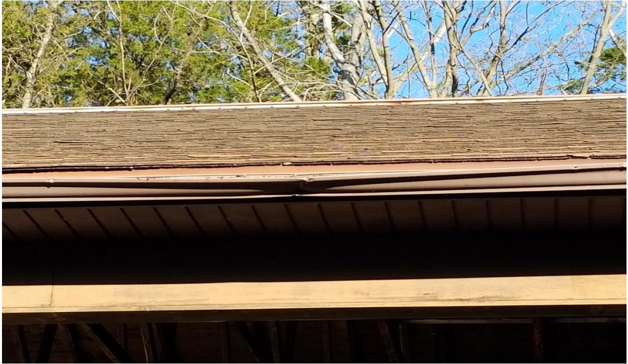
Existing conditions of roof shingles and failing gutters.
