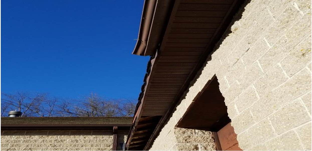
Missing soffit, gutters and deteriorated fascia.
