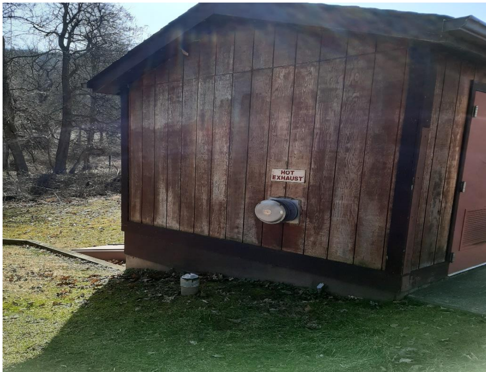
Composting Toilet System #1 PVC Sleeve for Grounding Rod
