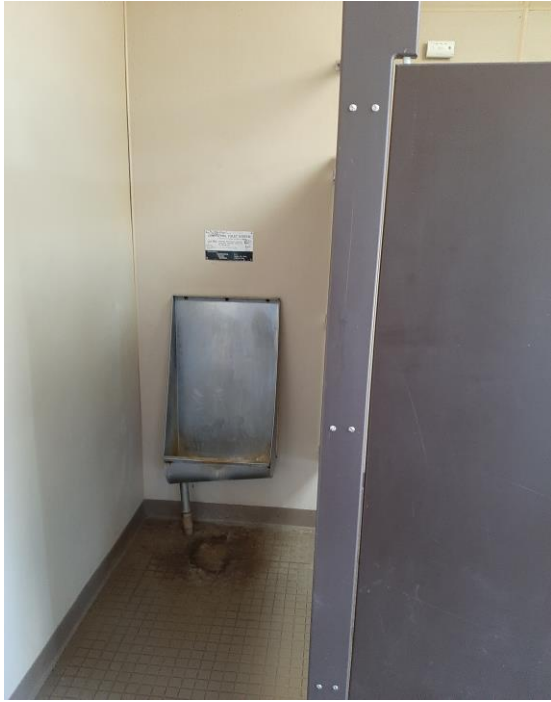
Composting Toilet System #1 Interior
