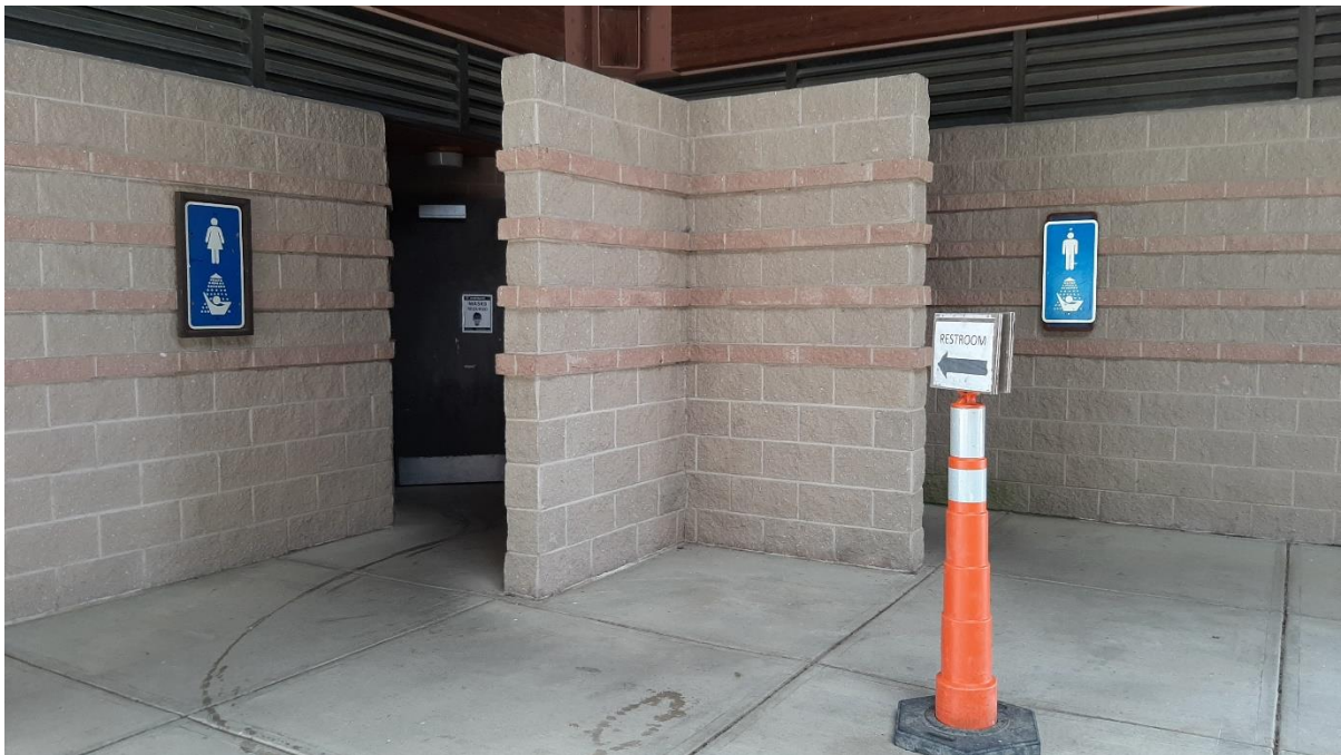
Existing Left Side Restroom Entrances from the Pavillion
