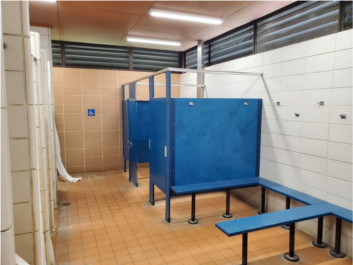
Existing Men's Restroom Interior.
