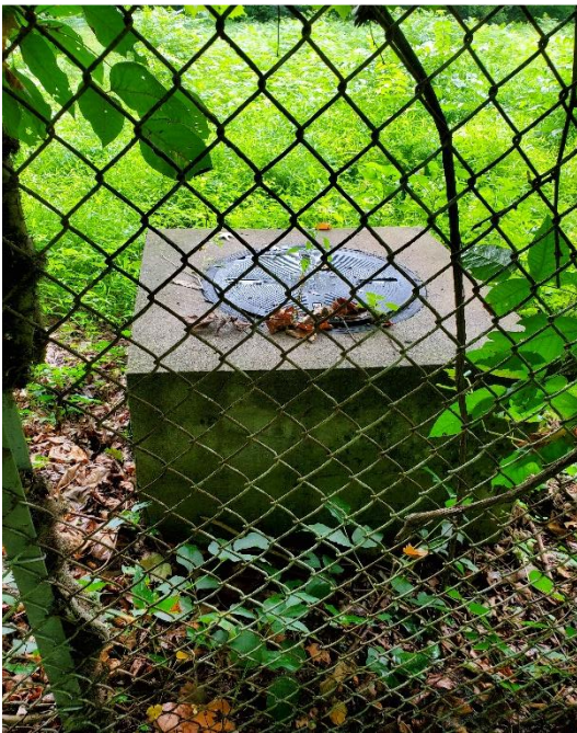
Existing fenced Leach Field across County Road 619.
