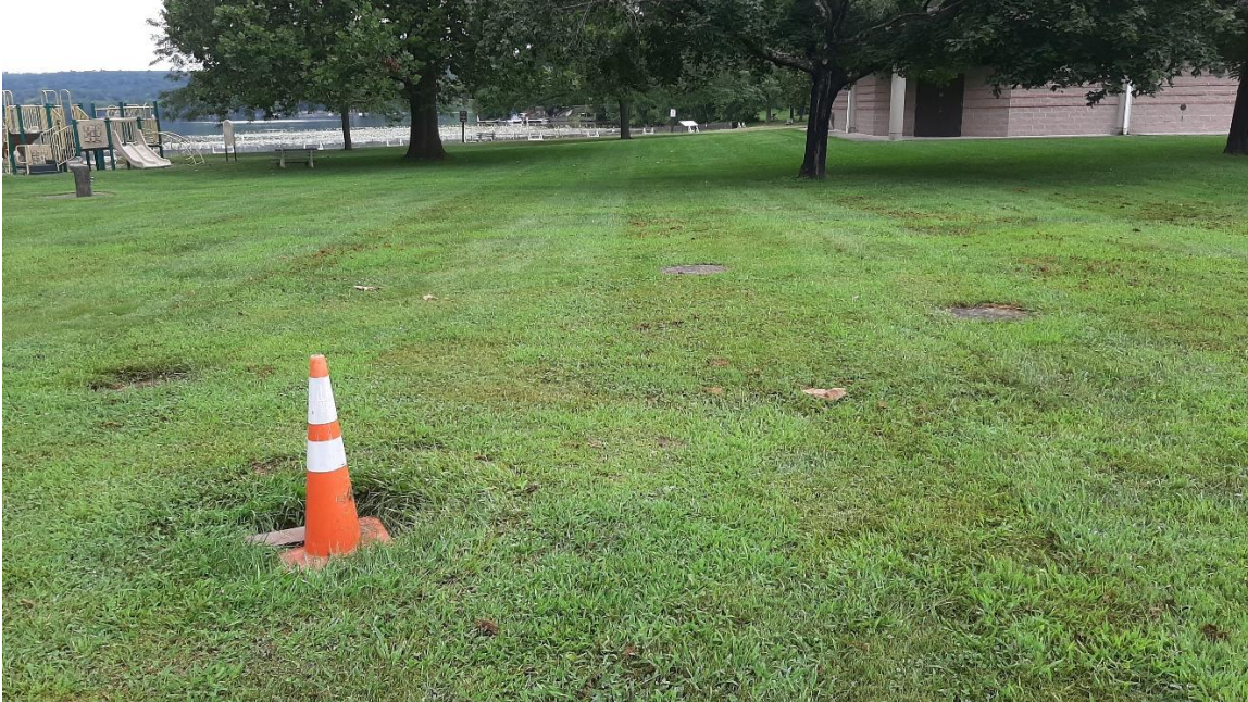
Location of the two septic underground holding tanks at the Pump House. Lines from the bathhouse to these tanks are gravity fed lines.
