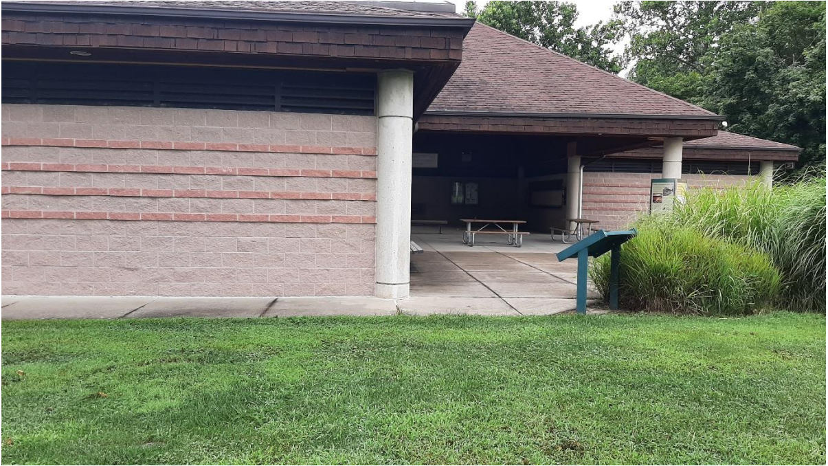
Existing Beach Bath House Exterior at Swartswood Lake
