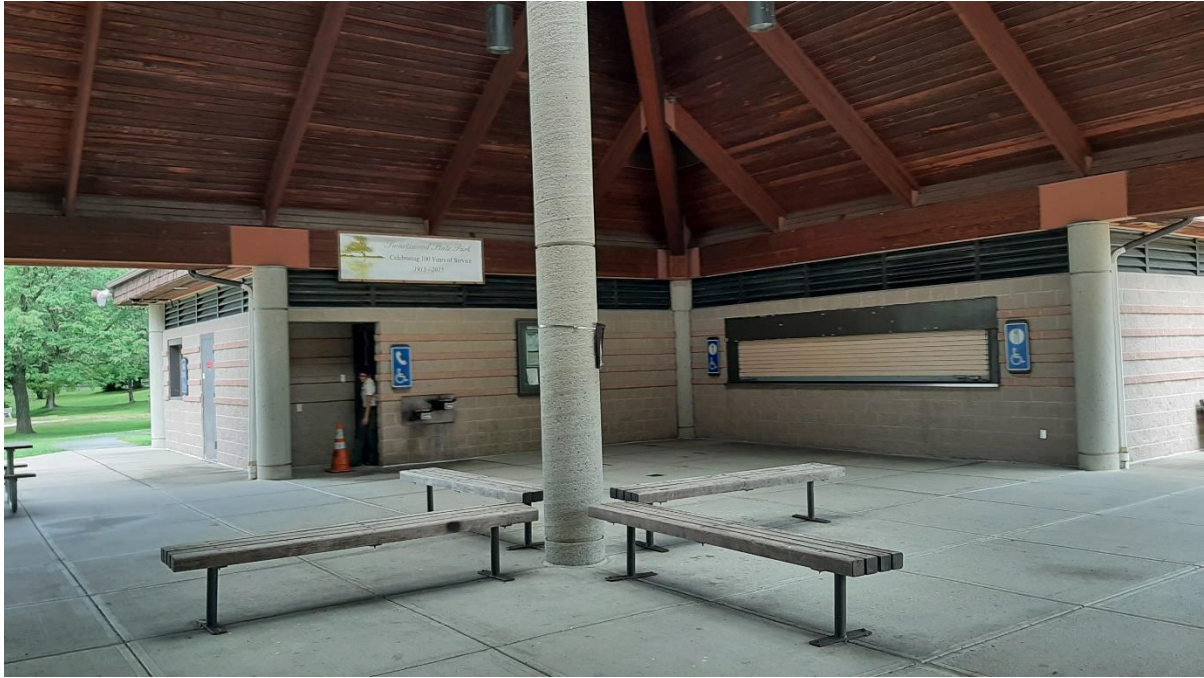
Existing Beach Bath House Connecting Pavillion
