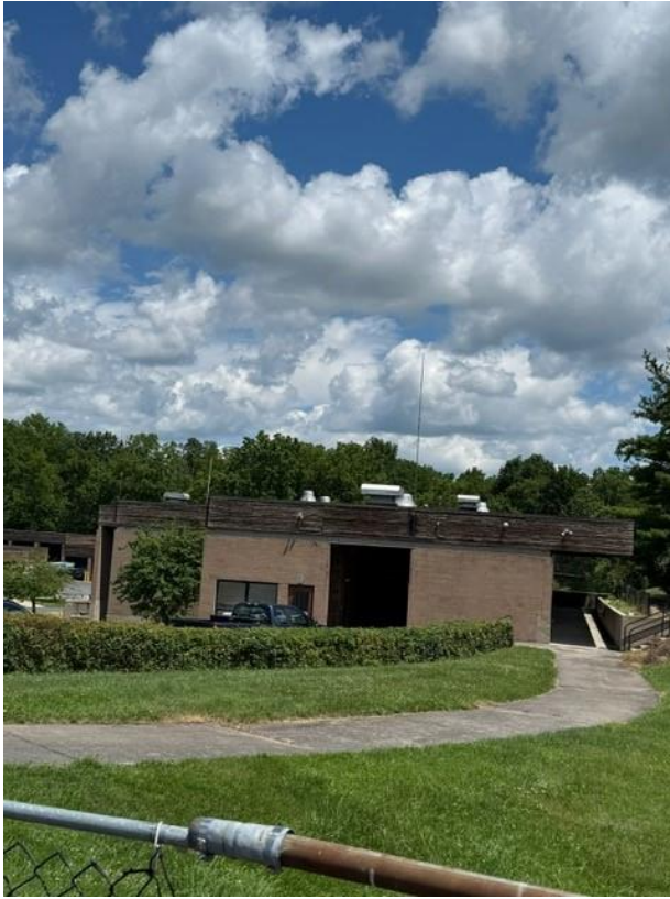
The Nursery building
