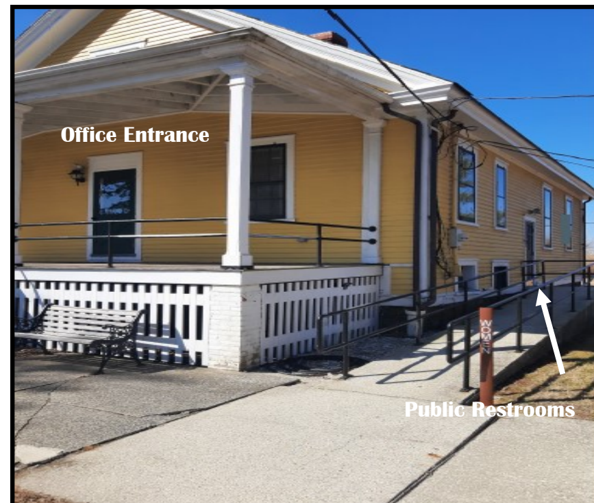
Photos Guardhouse - Exterior EXHIBIT 'C'
