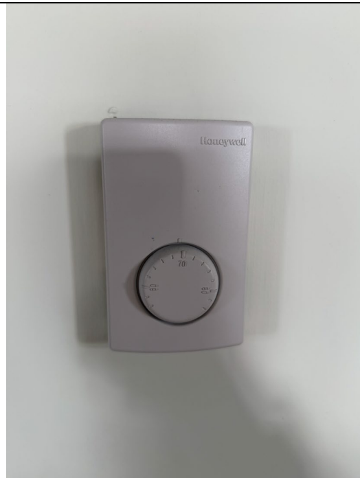
Picture 16: Typical manual thermostat
