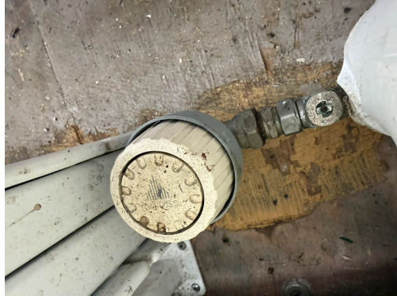
Picture 10: Typical fin tube radiator Danfoss valve
