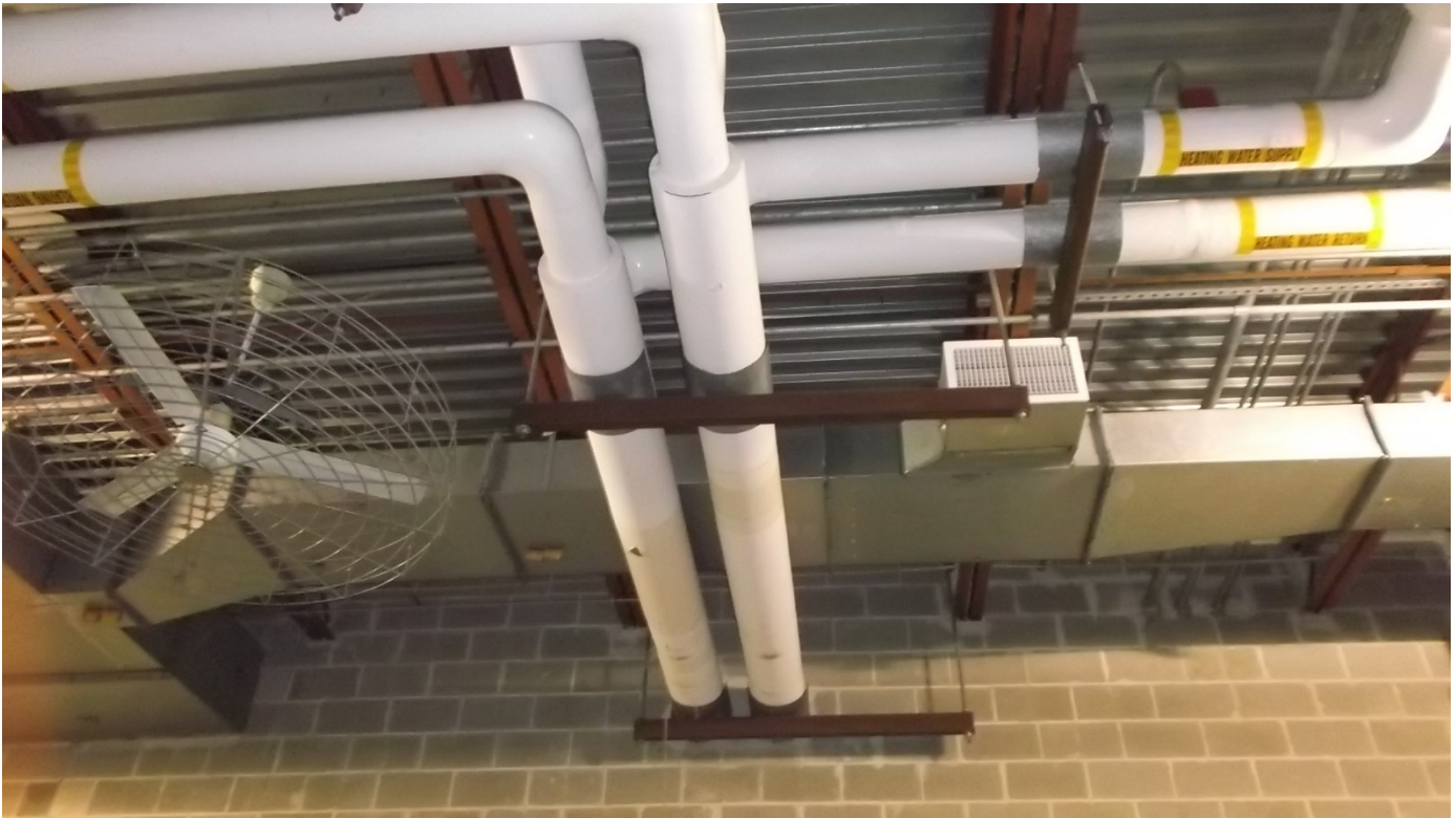
Heating water supply and return lines at wall just outside boiler room.
