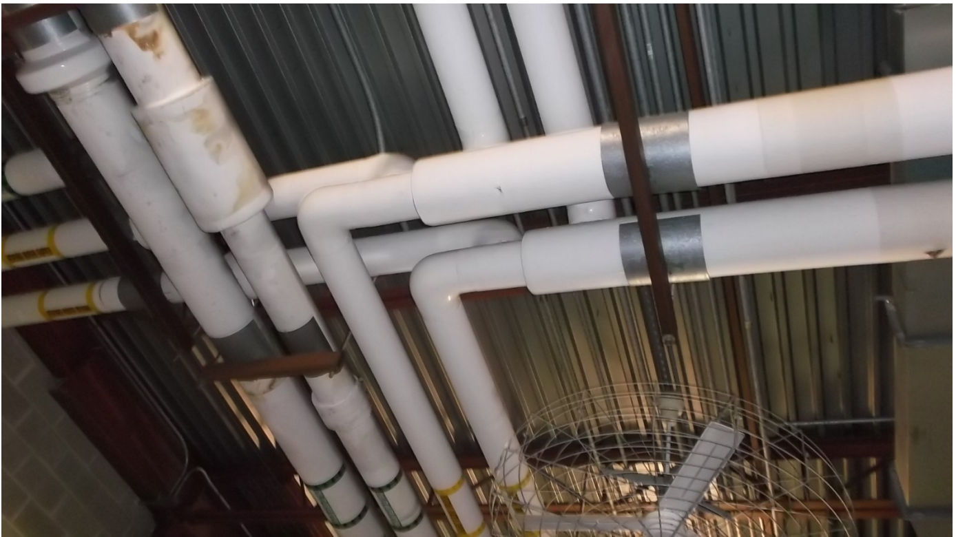
Heating water supply and return lines split into two branches in this area.
