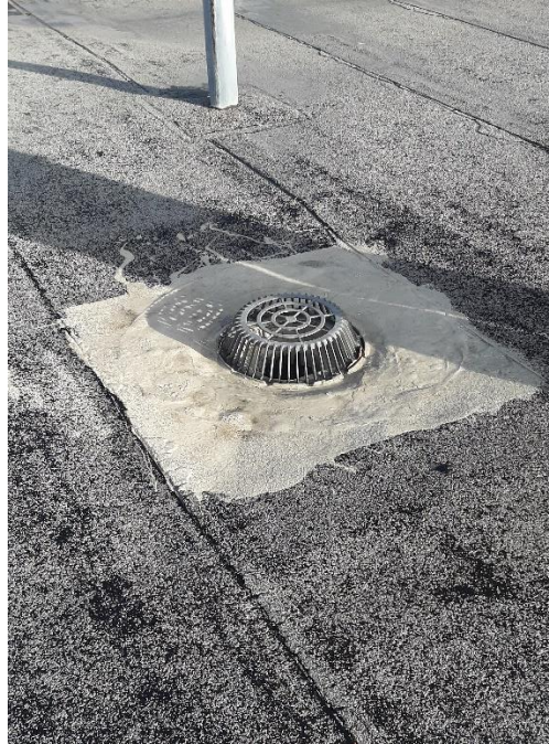
Existing condition of roof patch repair around the roof drains
