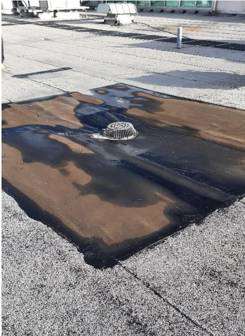
Existing condition of roof patch repair around the roof drains
