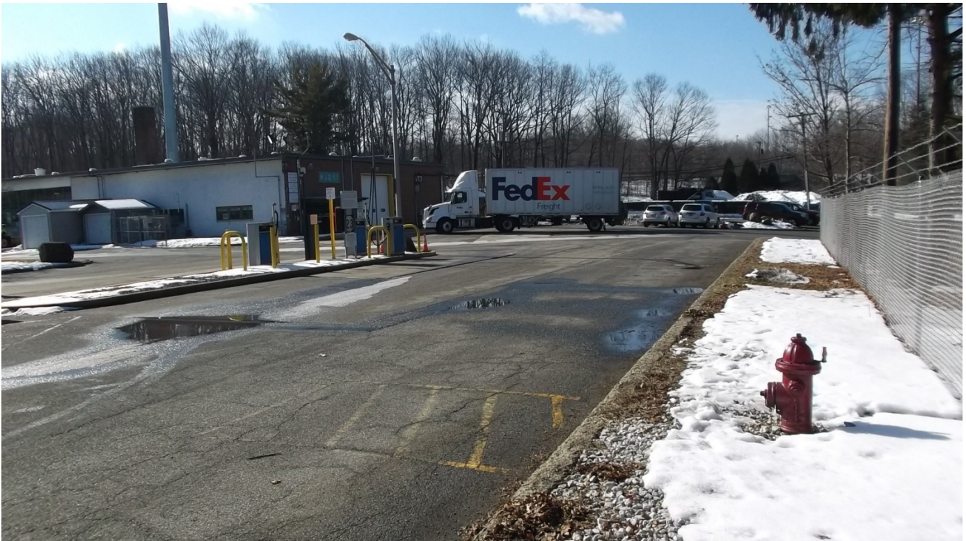
Existing fueling facility.
