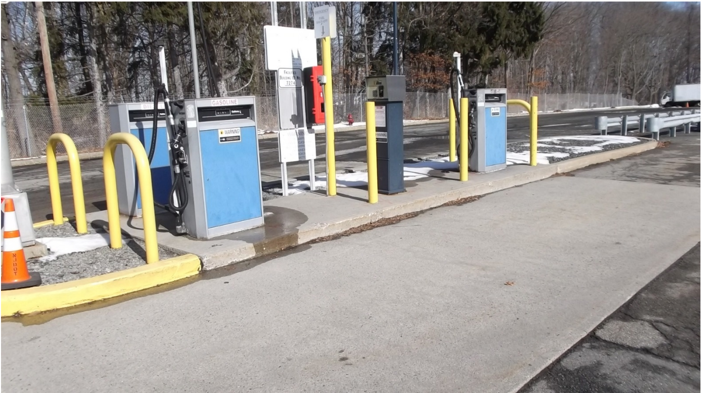
Existing dispensers to be demolished.
