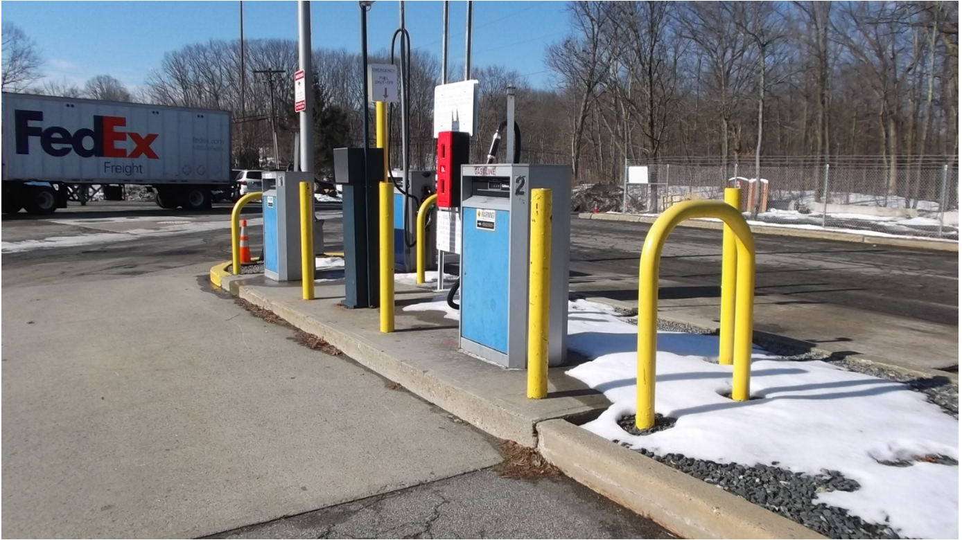
Existing dispensers to be demolished.
