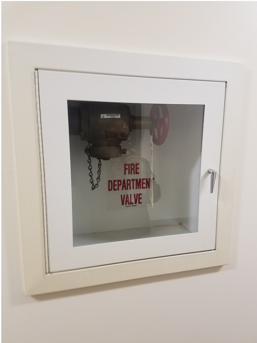
Fire Valve Cabinet (Typical) EXHIBIT 'C'
