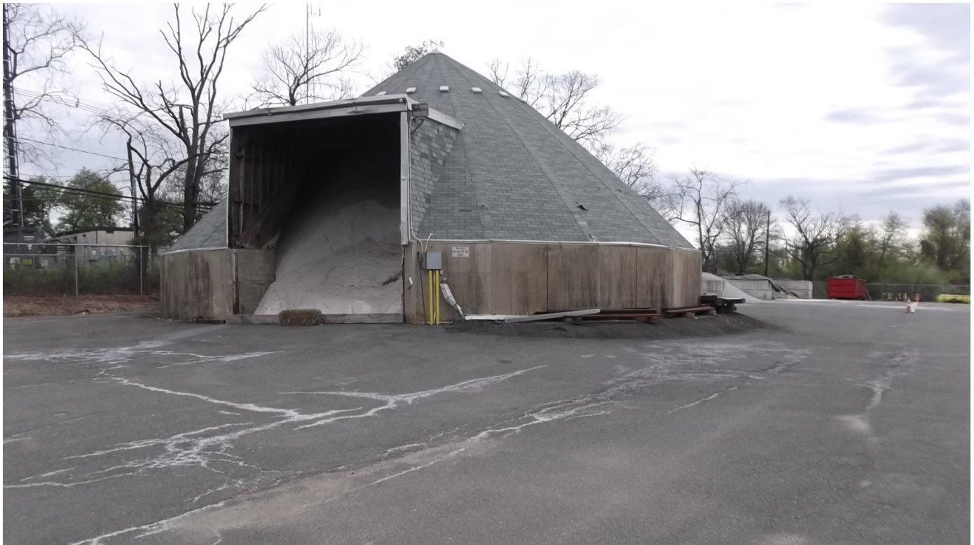
Salt Dome at DOT West Trenton Maintenance Yard
