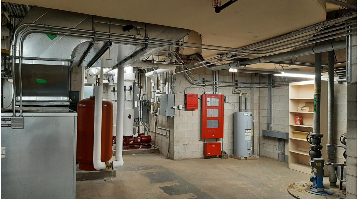
Existing Main Mechanical Room-Basement F&A Building
