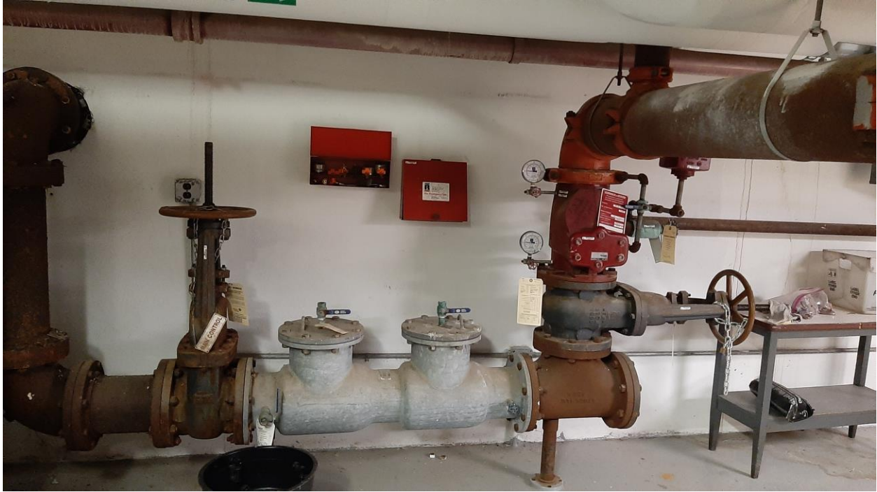
MOB Basement- Existing Partial Sprinkler System Water Main Control Valves.
