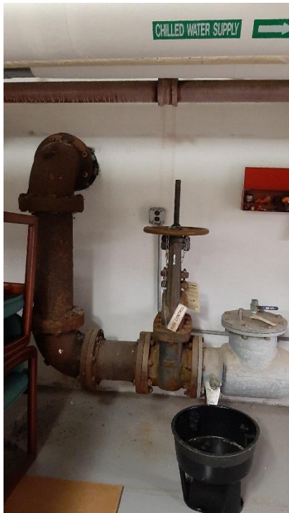
MOB Basement- Existing Backflow Preventor Valve
