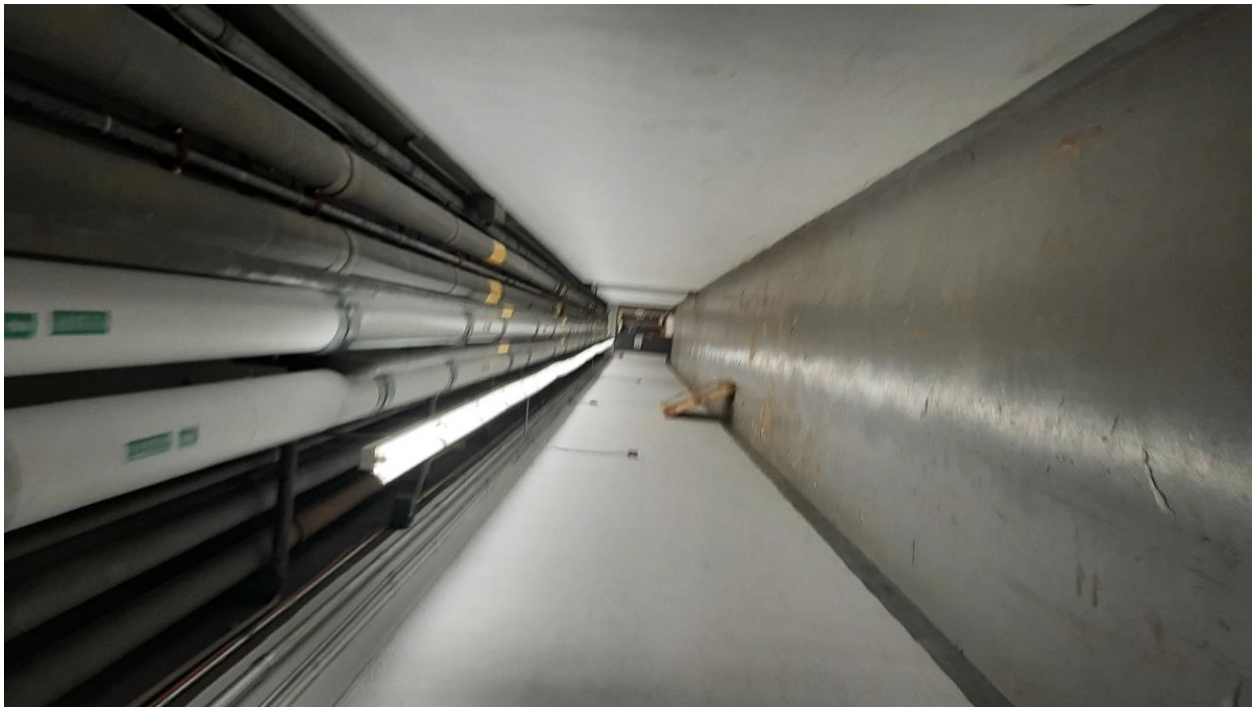
Existing Hallway Connecting MOB Basement and F&A Basement.
