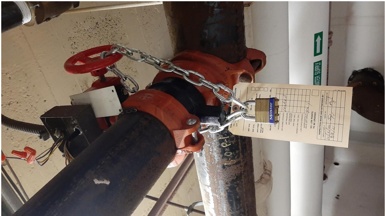
MOB Basement- Existing Partial Sprinkler System Water Main Control Valves.
