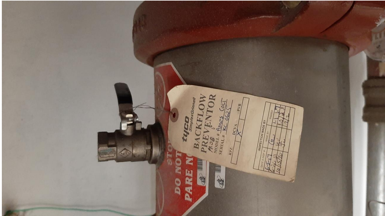
MOB Basement- Existing Backflow Preventor Valve
