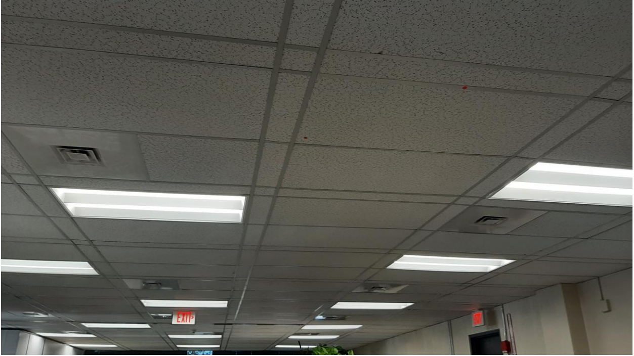
Existing First Floor Suspended Ceiling System, Exit Signs, Lighting Fixtures and Diffusers.
