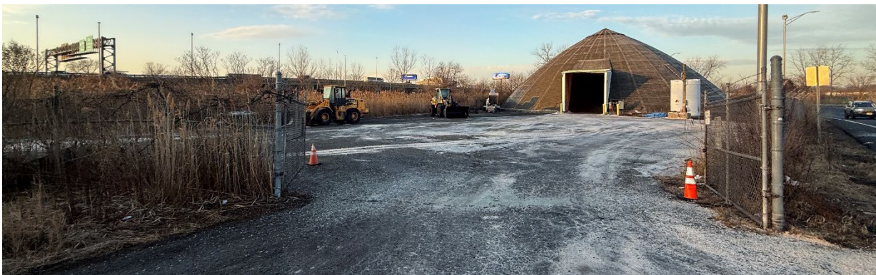
Overview from Entrance of Yard
