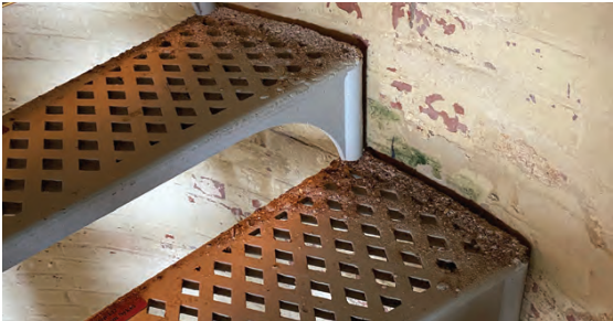
Spiral Cast Iron stairs, cantilevers from center column and has anchored in 1990's to the exterior wall every four treads. (05-1)
