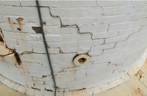
Through wall vent at watchtower level, and star cracking due to corrosion. (05-5)
