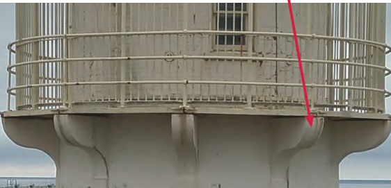
Watchtower Walkway supported by stone brackets below. (05-2) See stone brackets below.
