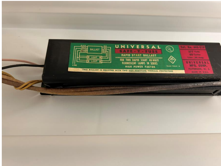
Photograph 5 – Light Ballast – Not Labelled Non-PCB
