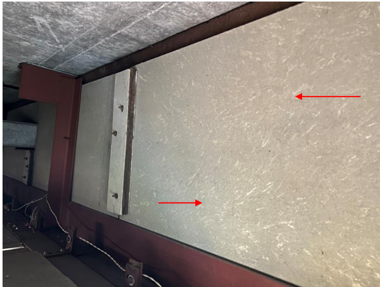
Photograph 3 – Cementitious Panel and associated Insulation along Perimeter Wall (Confirmed ACM/None Detected)
