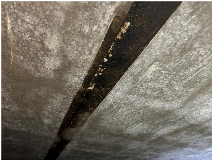
Photograph 2 – Sealant and Filler at Ceiling Concrete Joints (None Detected/None Detected)
