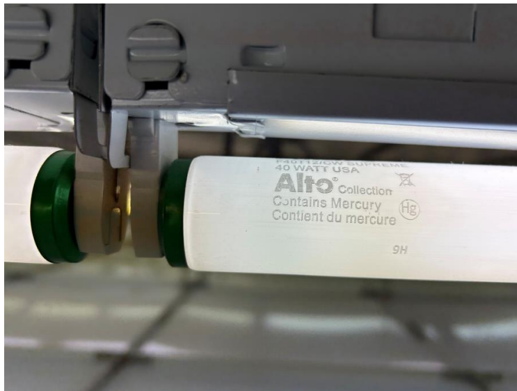
Photograph 6 – Fluorescent Bulb Mercury Containing Label
