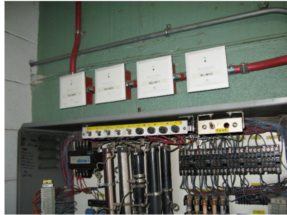
Photo #12 Notifier Fire Alarm Relays Elevator machine room.
