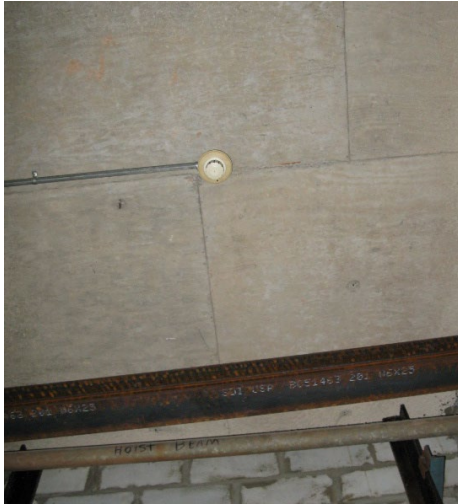
Photo #15 Smoke Detector Top of elevator hoistway.
