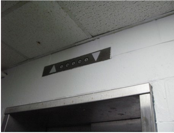
Photo #03 Hall Lanterns and Position Indicator Second level front.
