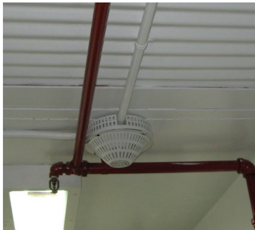
Photo #13 Heat Detector with Protective Cage Typical cell block elevator lobby.
