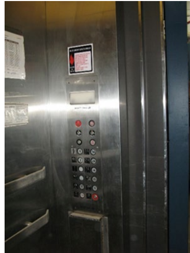
Photo #02 Elevator Control Panel Cab front wall.
