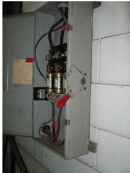
Photo #10 Elevator Disconnect Switch Needs cleaning.
