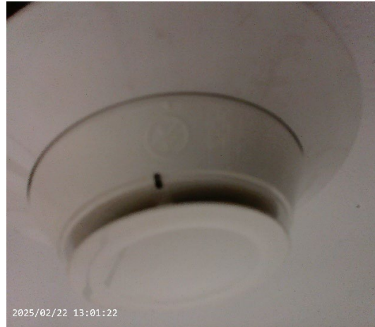
Photo #14 Smoke Detector Typical in main corridor.
