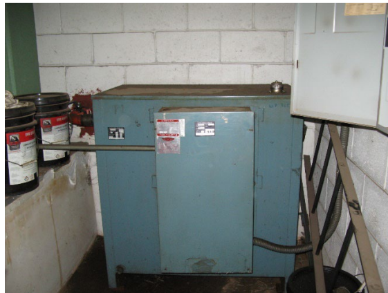
Photo #08 Hydraulic Power Unit Water has penetrated this equipment.
