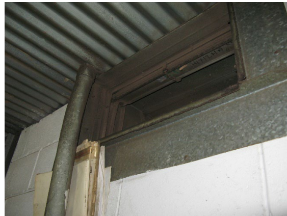
Photo #B16 Fire Damper AC duct into elevator machine room.
